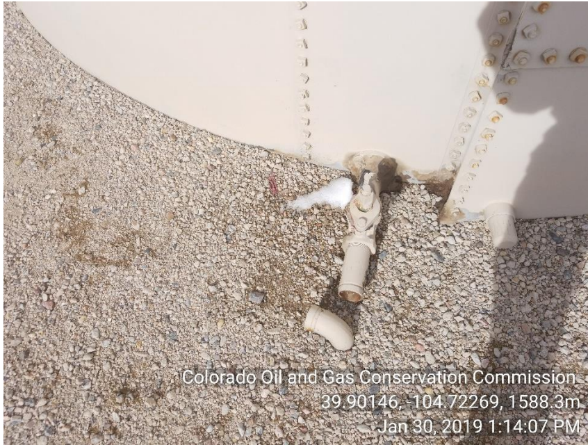
Photo 3 load line to west crude oil tank not capped or plugged.
