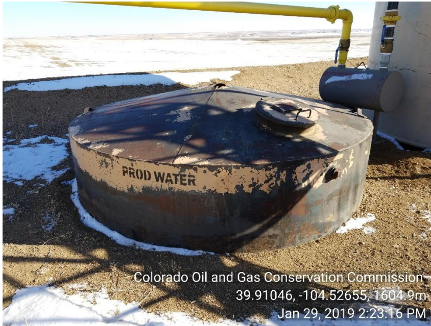
Photo 3 Produced water tank no placards or volume
