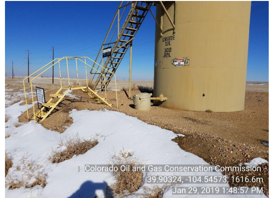
Photo 4 TNK BTYR inadequate berms
