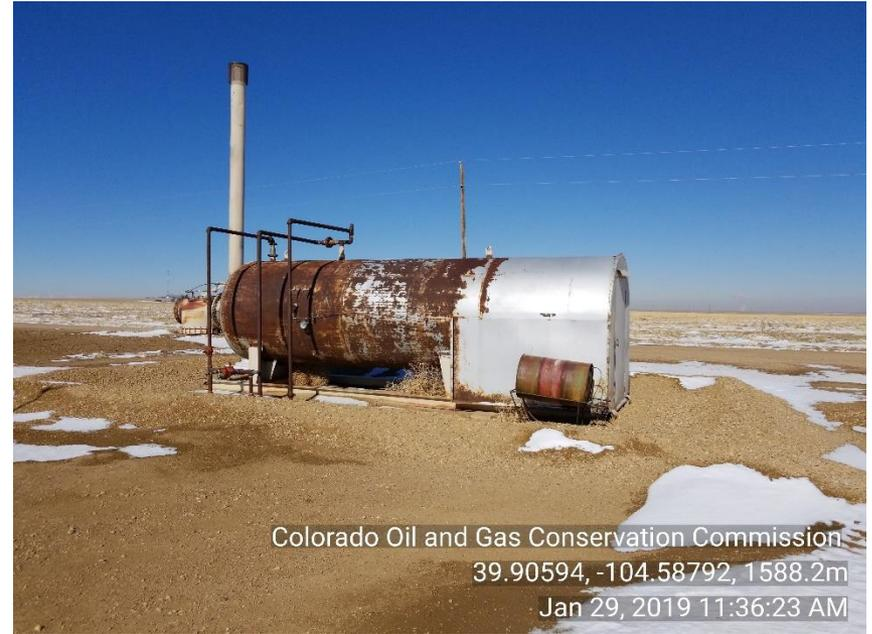
**Photo 3 TNK BTRY trach (roll of cable) tank not painted**
