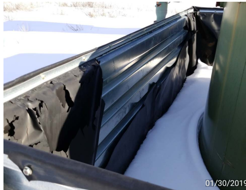
Photo 2. Tank liner is torn.
