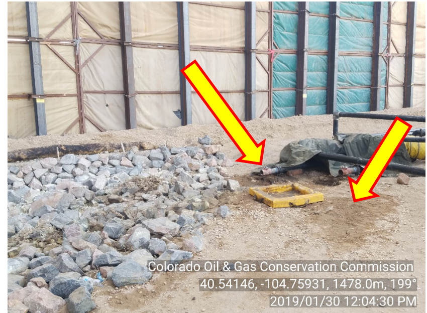
Photo #2 G & D Hanks /27-N Pad Stained soil - Condensate
