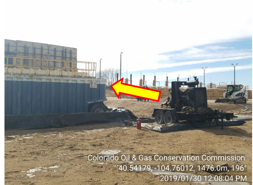
Photo #4 G & D Hanks /27-N Pad Internal combustion Transfer pump Close proximity to hydrocarbon tanks ≈ 15 feet
