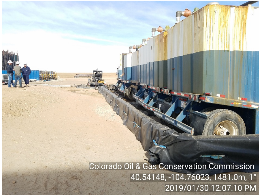
Photo #3 G & D Hanks /27-N Pad Flowback tanks – NOT grounded
