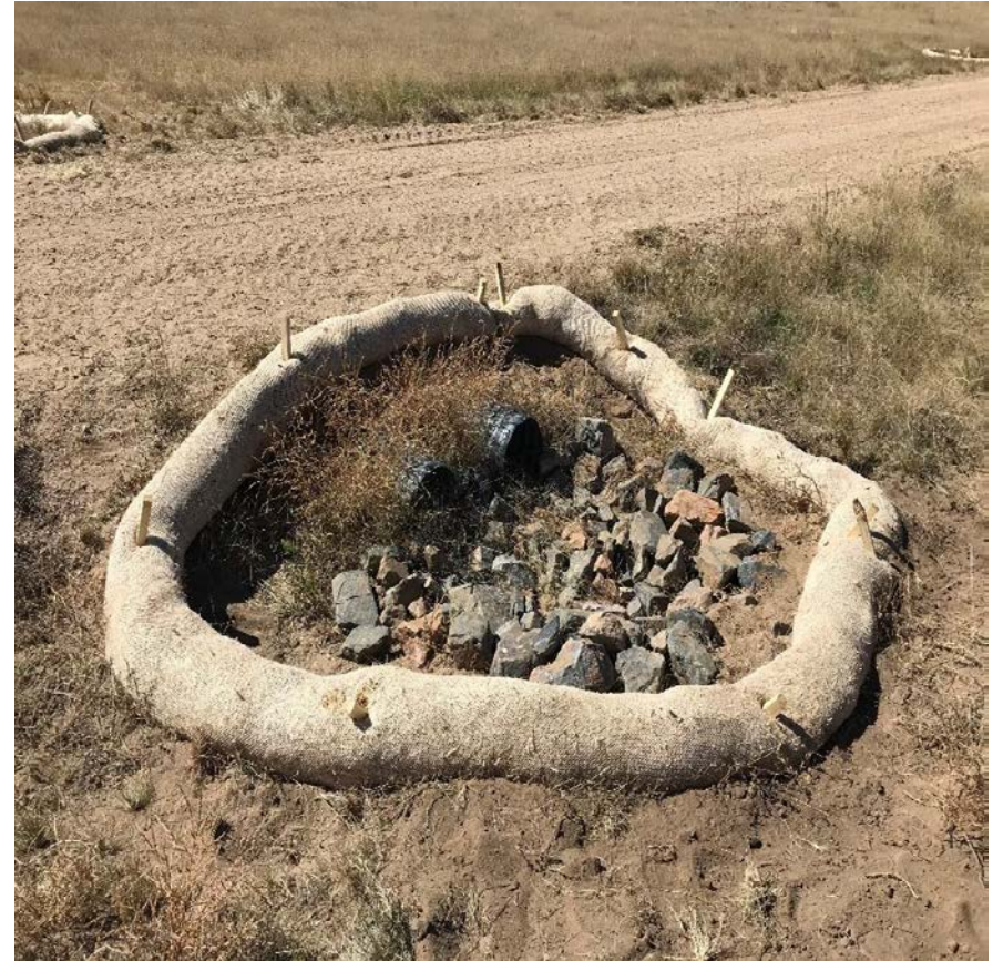
10/3/18 - LTE/Hilcorp Photograph 8: Sediment has been removed. Inlet and outlet protection have been added to all 3 culvert locations.
