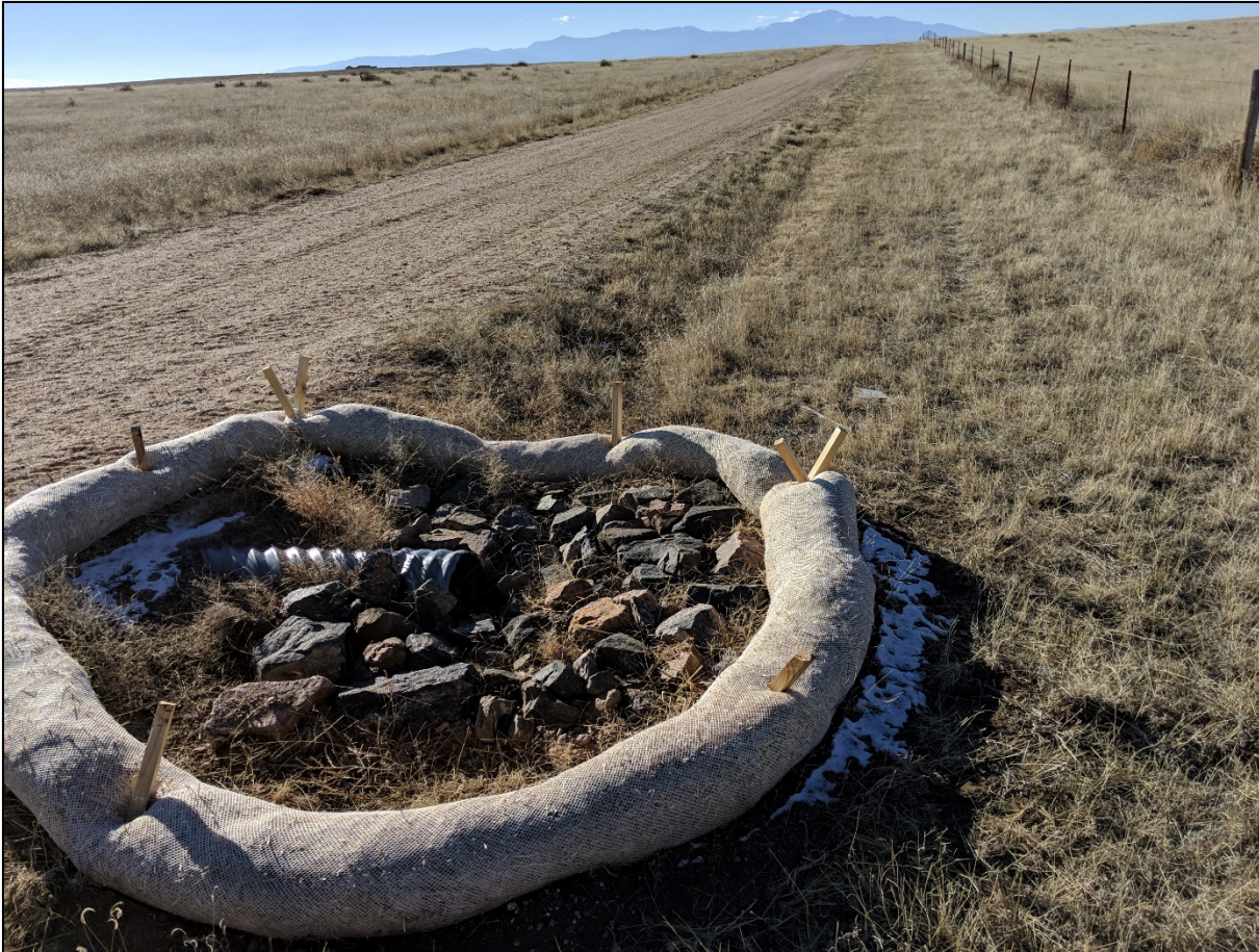
Photo 7. The inlet culvert. Water flows from the east and the west to the culverts. Rock rip/rap is improperly installed as it is piled too high in front of the culvert which appear to be restricting water flow. The wattles are temporary BMP's and are not a long term solution. A long term solution could be sediment traps and rock check dams.
