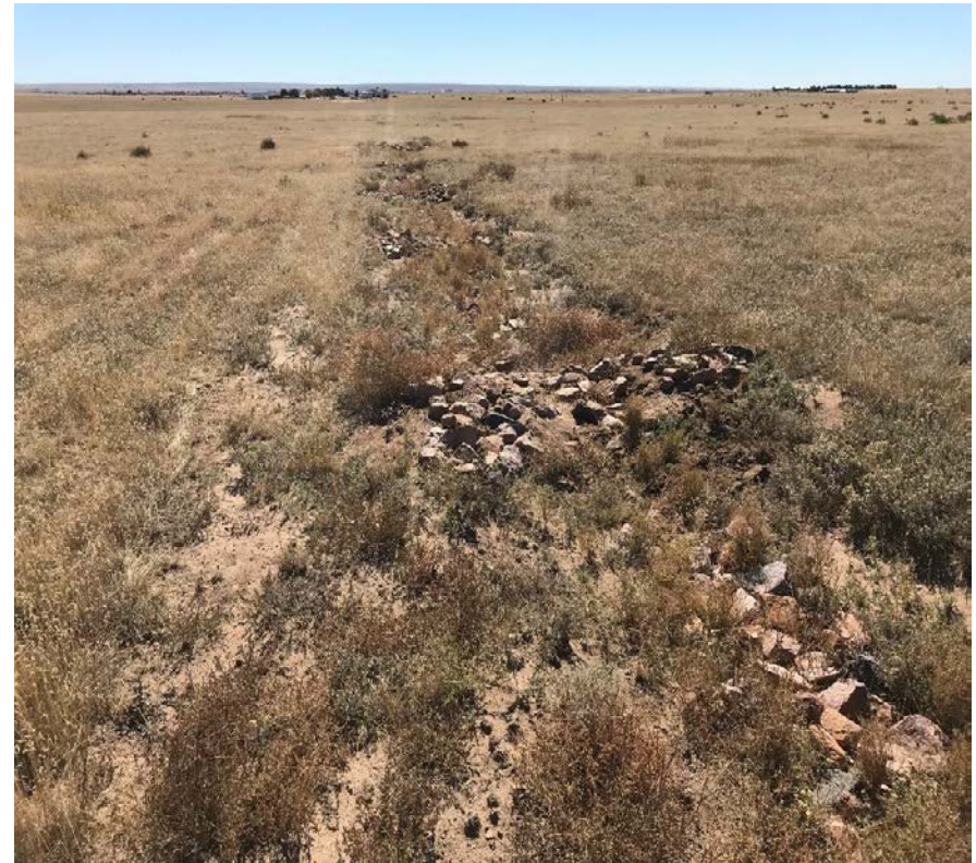
10/3/18 - LTE/ Hilcorp Photograph 3: Corresponds to COGCC inspection photo 7. Check dams have been repaired. Old sandbags have been removed and vegetation is filling in.
