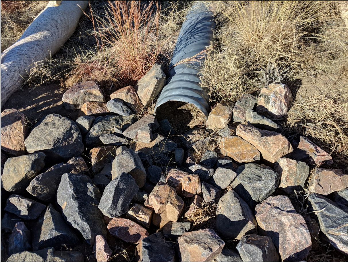
Photo 10. Sediment remains in the culvert. Rock rip/rap is improperly installed as it is piled too high in front of the culvert which appears to be restricting water flow.
