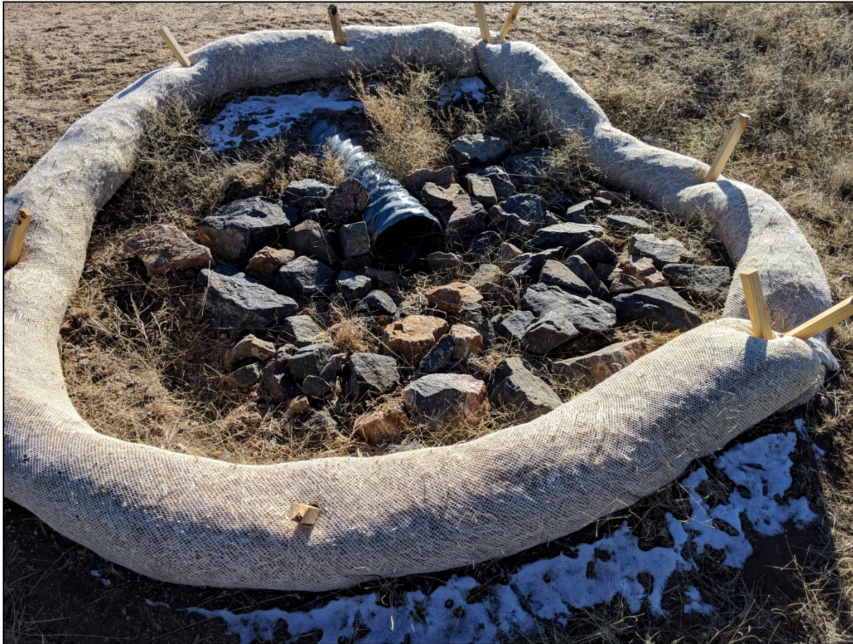
Photo 8. The inlet culvert. Rock rip/rap is improperly installed as it is piled too high in front of the culvert which appear to be restricting water flow. The wattles are temporary BMP's and are not a long term solution. All culverts need to have long term sediment controls.
