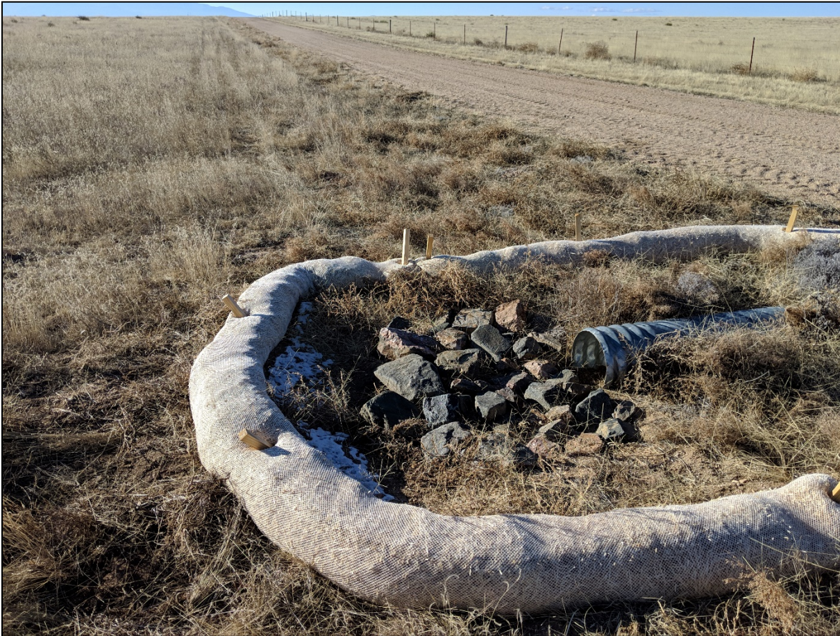
Photo 9. The outlet culvert. Rock rip/rap is improperly installed as it is piled too high in front of the culvert which appear to be restricting water flow. The wattles are temporary BMP's and are not a long term solution. All culverts need to have long term sediment controls.
