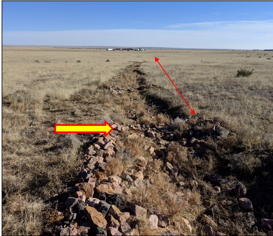
COGCC Photo 2. The drainage channel extends far out into the pasture. This is additional disturbance caused by erosion. The channel needs to be recontoured to grade and reclaimed/reseeded along the red arrow to the yellow arrow. A proper sediment trap should be constructed at the yellow arrow.
