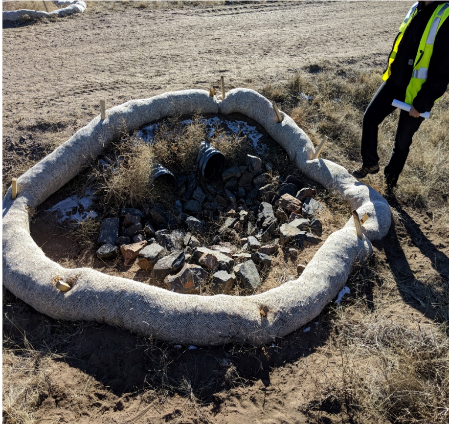
COGCC Photo 6. The inlet culvert. Rock rip/rap is improperly installed as it is piled too high in front of the culvert which appear to be restricting water flow. The wattles are temporary BMP's and are not a long term solution. A long term solution could be sediment traps and rock check dams.
