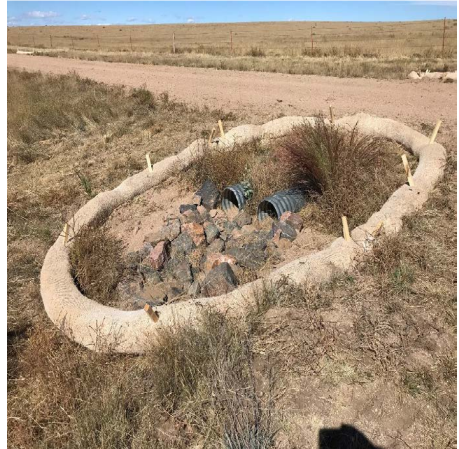
10/3/18 - LTE/ Hilcorp Photograph 7: Corresponds to COGCC inspection photo 12. Sediment has been removed. Inlet and outlet protection have been added.
