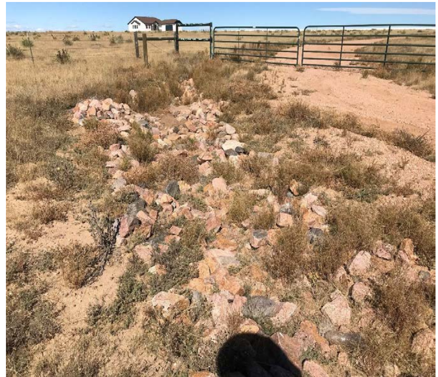
10-3-18 - LTE/Hilcorp Photograph 2: Corresponds to COGCC inspection photo 5. Erosion has been repaired and vegetation is filling in to stabilize.
