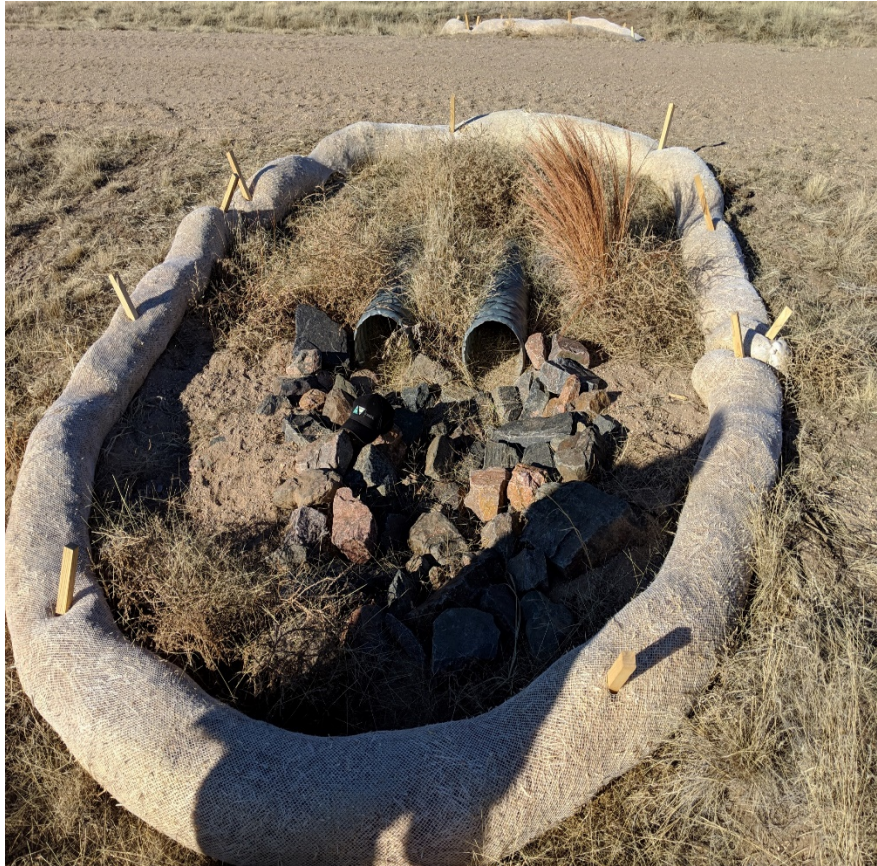
COGCC Photo 5. The outlet culvert. Rock rip/rap is improperly installed as it is piled too high in front of the culvert which appear to be restricting water flow. The wattles are temporary BMP's and are not a long term solution.
