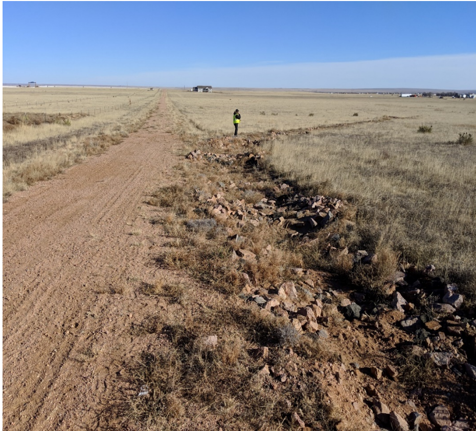
COGCC Photo 1. Facing east on the access road. Rock rip/rap can be seen in the drainage channel. Rock check dams have been lowered to allow water flow per previous inspection. See further information on photo 2.
