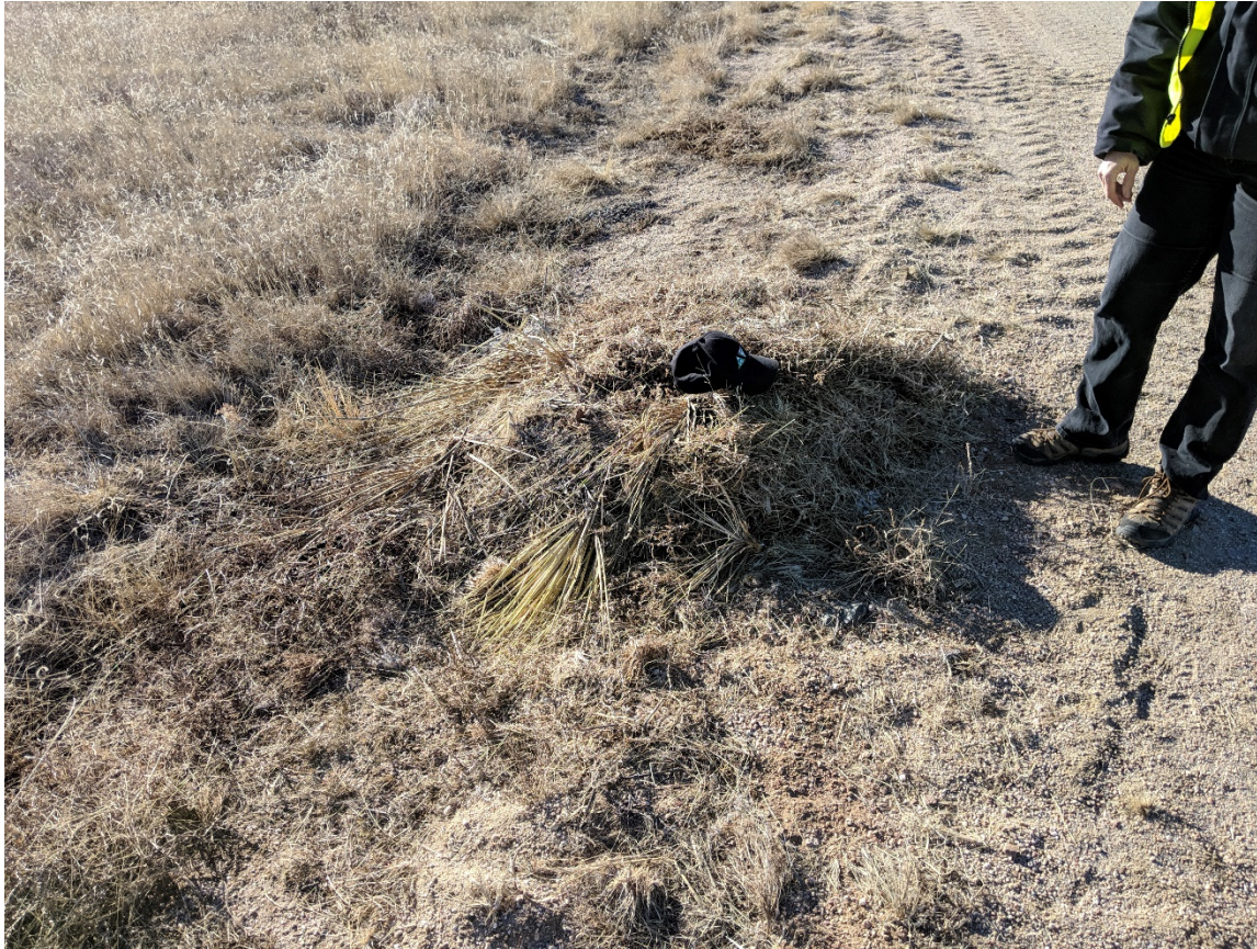
Photo 11. Piles of debris were found along the access road. It appears seeding operations dragged debris into piles. The debris piles need to be removed.
