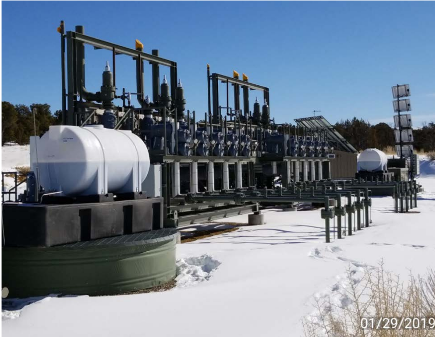
Photo 5. Well head manifold.
