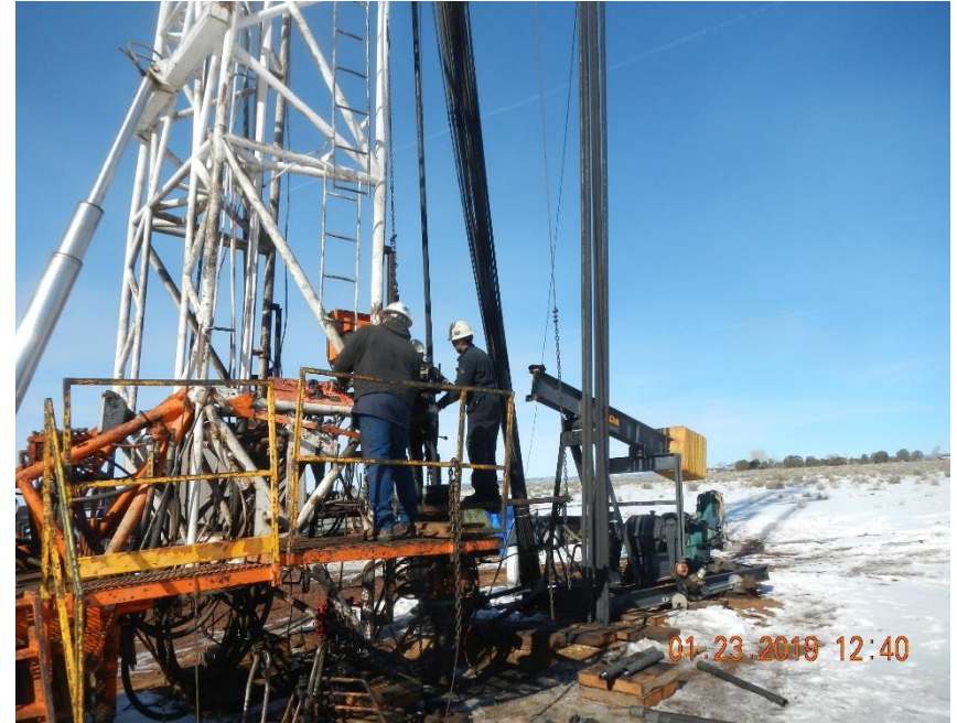
Tripping in hole in preparations for MIT.
