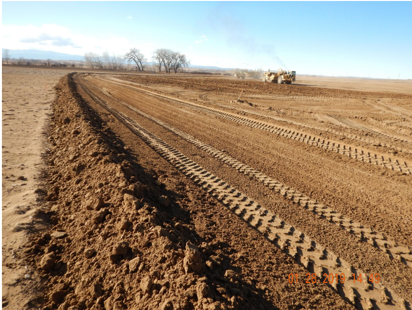
Photo 3. Photo taken from the southern perimeter of the location, facing West. Photo illustrates a temporary BMP (ditch). BMP has not been properly stabilized as unconsolidated soil material is not a properly functioning BMP. Unconsolidated soil material becomes a potential pollutant itself and is susceptible to wind and water erosion. Note: Per Rule 805.c., Operator shall control fugitive dust caused by their operations.
