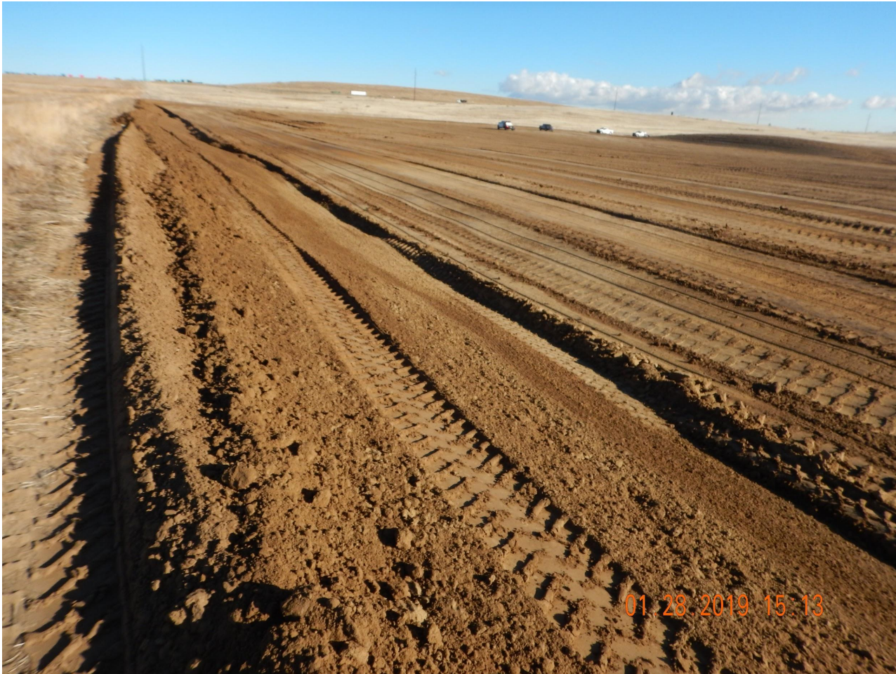
Photo 7. Photo taken from the northern perimeter of the location, facing East. See comments under Photo 3. Note: Photo also illustrates the subsoil layer coloration indicating that topsoil has been salvaged to the appropriate depth.
