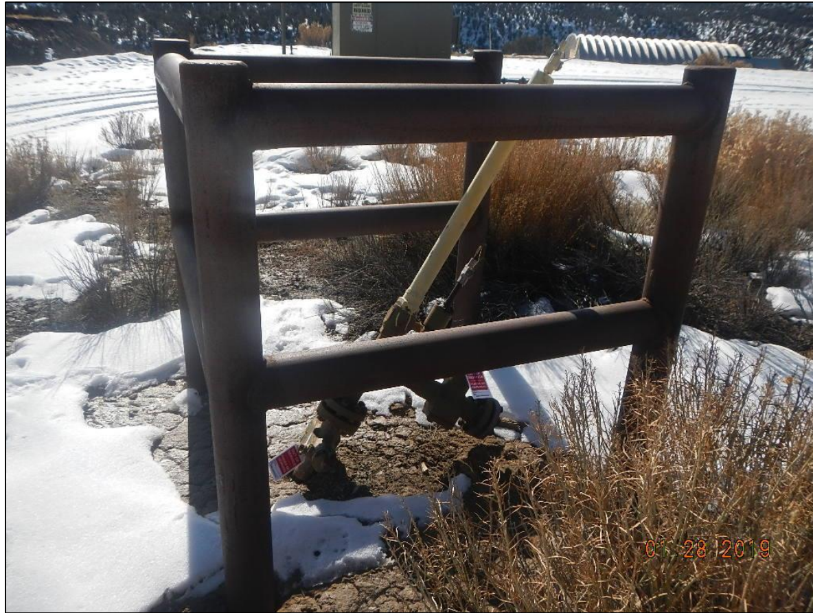
Riser locked out and tagged
