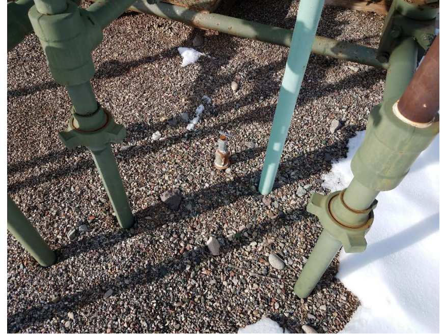
Location Photo #2, Unmarked, unused flowline riser.
