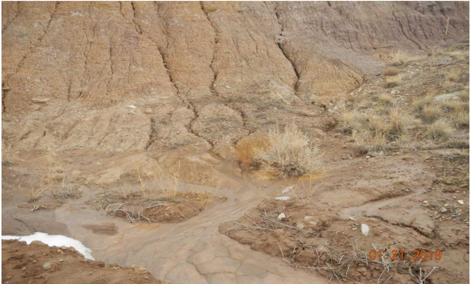
Photo#4: Erosion is occurring on & sediment migration off, of Cut slope.
