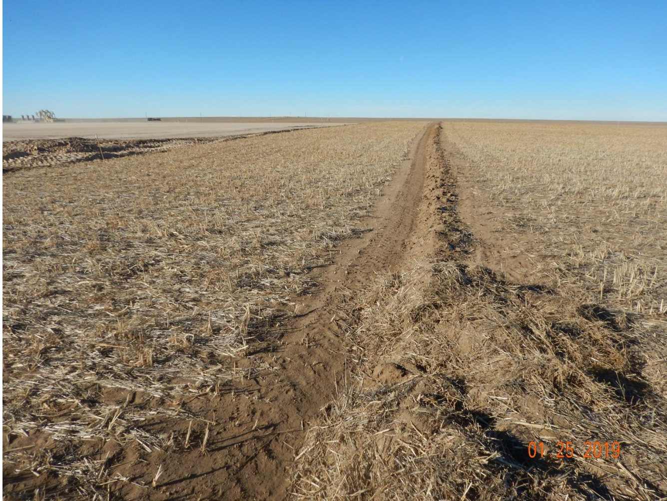
Photo 8: Photo taken from the northeast corner of the location, facing west. Photo shows ditch/berm BMP along perimeter of the location. See comments under photo 2.
