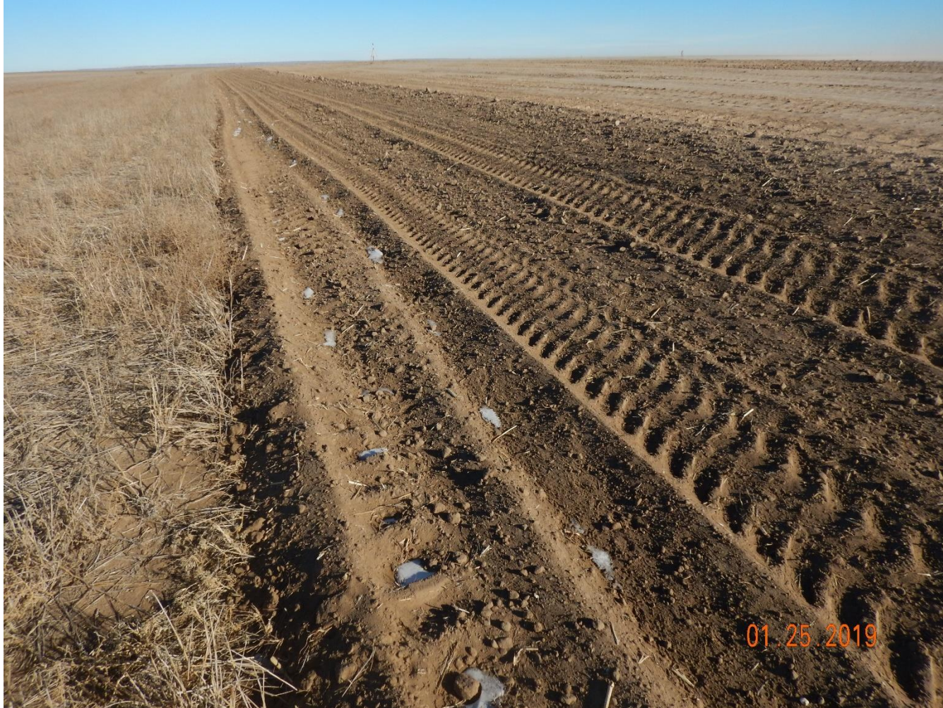
Photo 27: Photo taken from the west end of the topsoil stockpile, facing northeast. Photos shows topsoil stockpile has not been stabilized and remains loose material, and sufficient stormwater and erosion control BMPs do not appear to have been installed.
