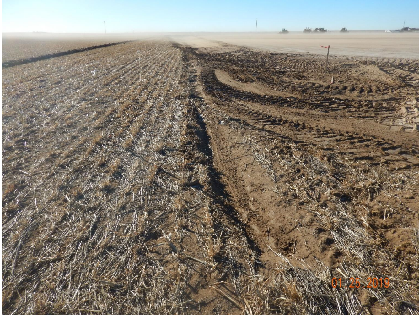
Photo 28: Photo taken from the northeast corner of the pad, facing south. Sufficient stormwater and erosion control BMPs do not appear to have been installed on the northeast corner of the pad. See comments under photo 11.
