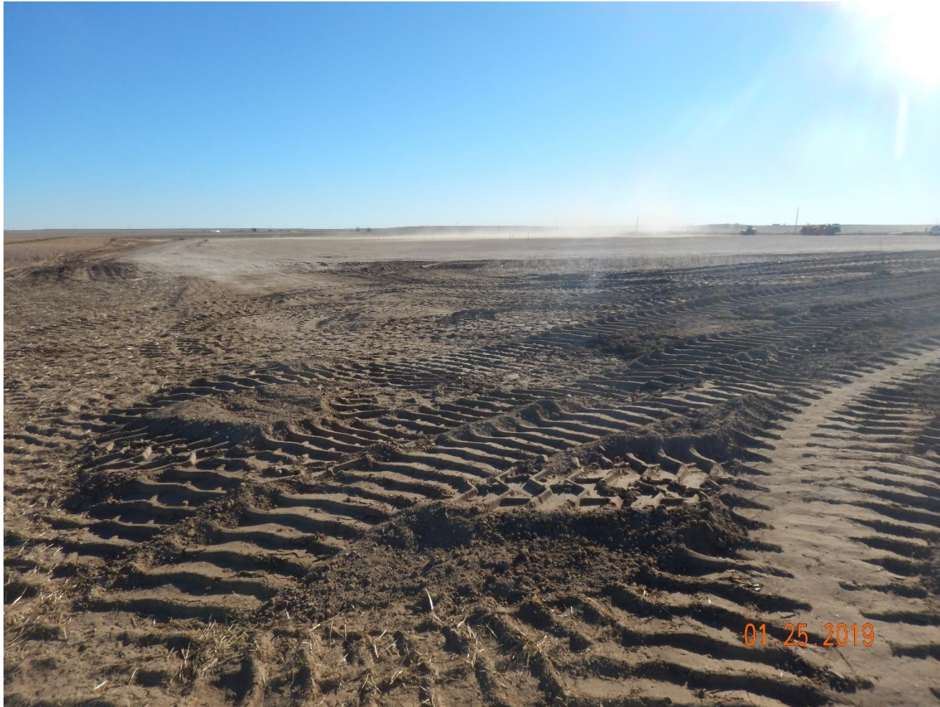
Photo 14: Photo taken from the northwest corner of the pad, facing southeast. Sufficient stormwater and erosion control BMPs do not appear to have been installed on the northeast corner of the pad. See comments under photo 11.
