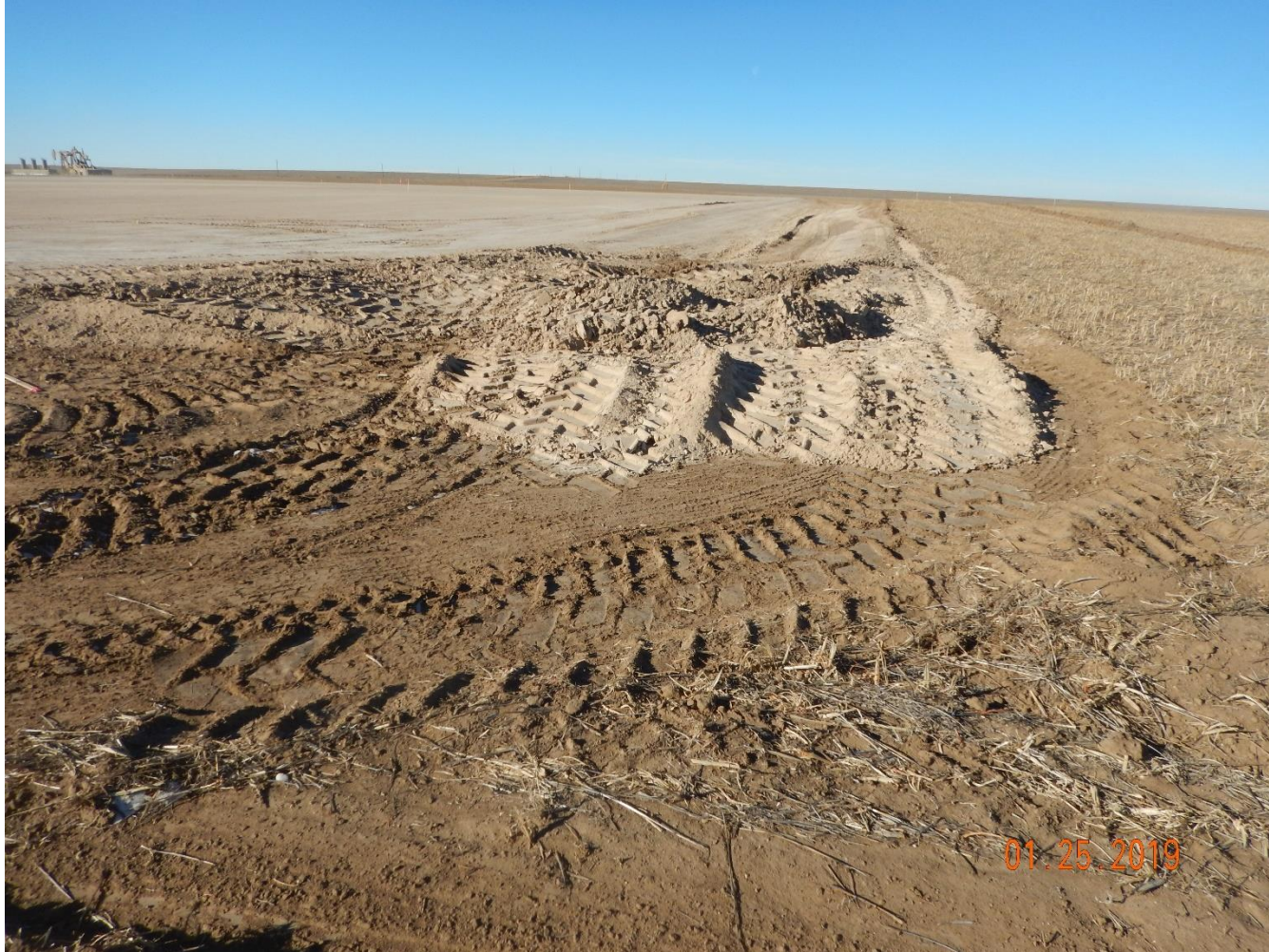
Photo 29: Photo taken from the northeast corner of the pad, facing east. Sufficient stormwater and erosion control BMPs do not appear to have been installed on the northeast corner of the pad. See comments under photo 11.
