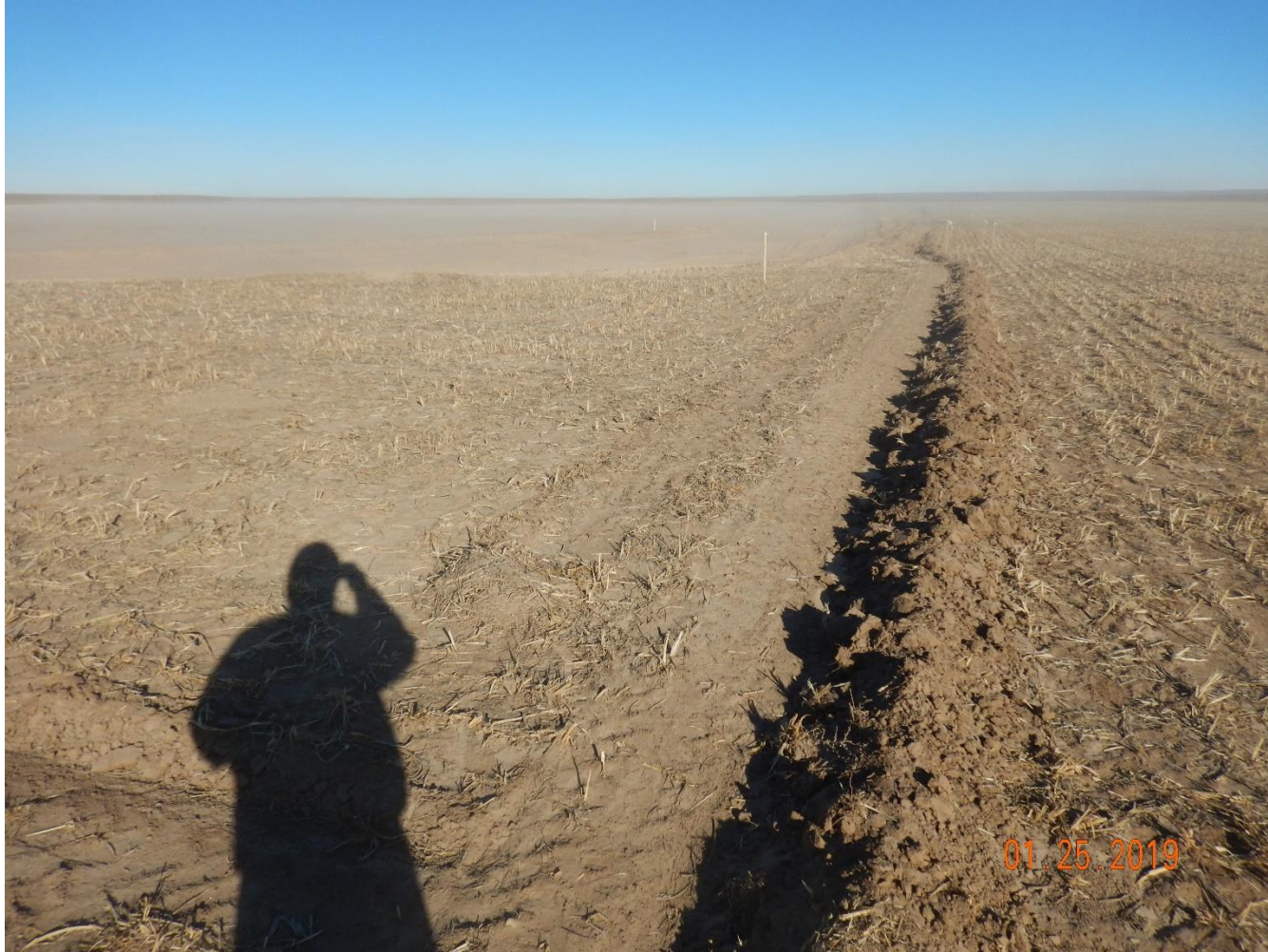
Photo 10: Photo taken from the southeast corner of the location, facing north. Photo shows ditch/berm BMP along perimeter of the location. See comments under photo 2
