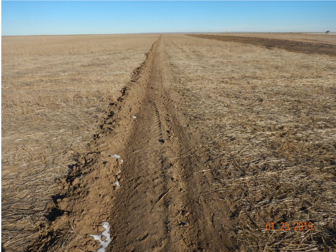
Photo 2: Photo taken from the southwest corner of the disturbance area, facing north. Operator appears to have installed a stormwater ditch and berm BMP along the perimeter of the disturbance area. Ditch/Berm BMP is shallow with unconsolidated material. Ditch/Berm BMP does not appear to have been constructed in accordance with good engineering practices, is improper and insufficient.
