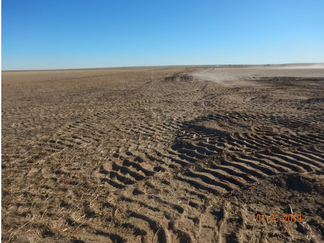
Photo 13: Photo taken from the northwest corner of the pad, facing east. Sufficient stormwater and erosion control BMPs do not appear to have been installed on the northeast corner of the pad. See comments under photo 11.
