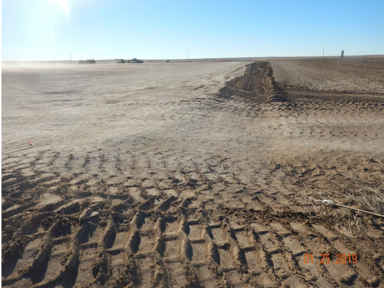
Photo 17: Photo taken from the northwest corner of the pad, facing south. Sufficient stormwater and erosion control BMPs do not appear to have been installed on the northwest corner of the pad. See comments under photo 11.
