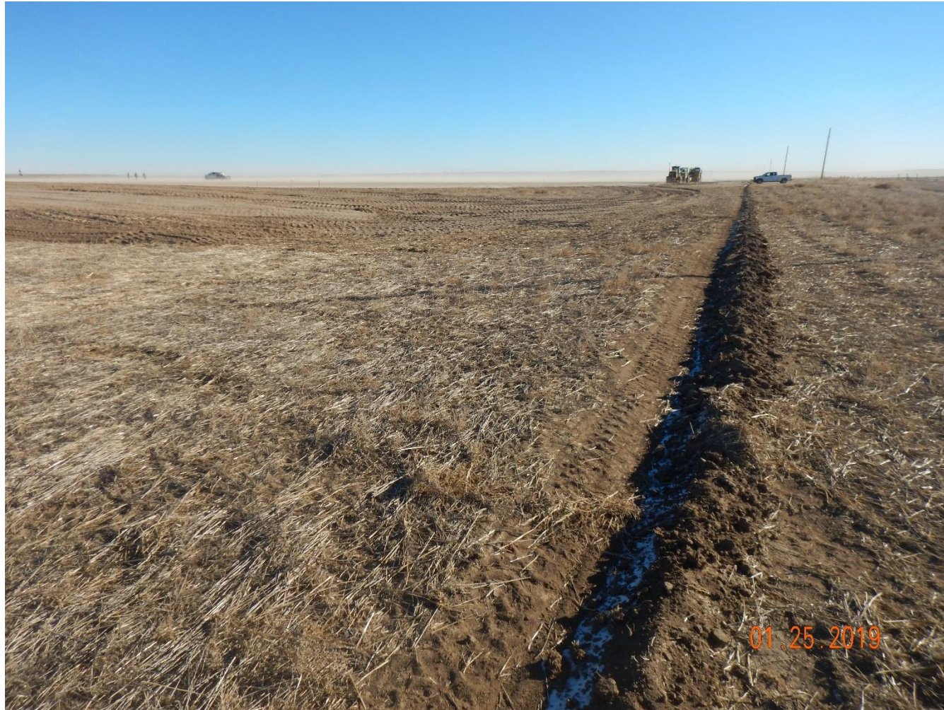
Photo 3: Photo taken from the southwest corner of the disturbance area, facing east. Photo shows ditch/berm BMP along perimeter of the location. See comments under photo 2.
