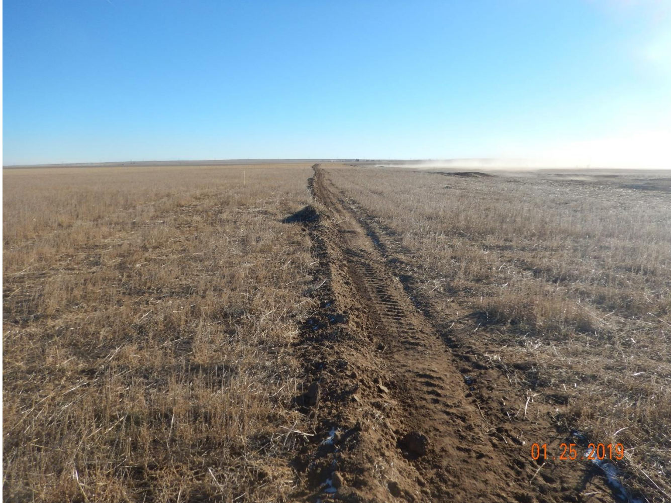
Photo 7: Photo taken from the northwest corner of the location, facing east. Photo shows ditch/berm BMP along perimeter of the location. See comments under photo 2.
