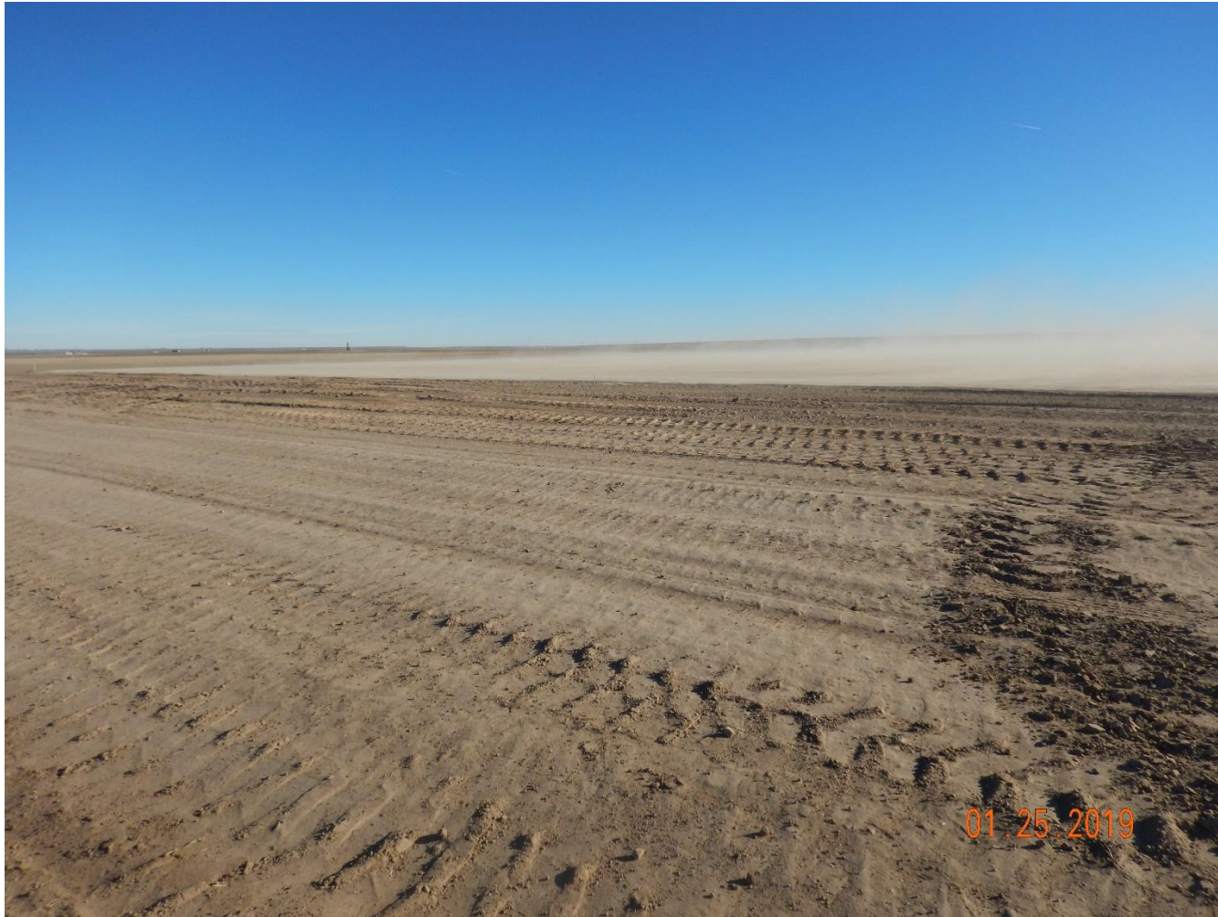
Photo 36: Photo taken from the west end of the location, facing northeast. Photo shows wind erosion transporting sediment offsite. This does not comport with rule 1002.e and 1002.f
