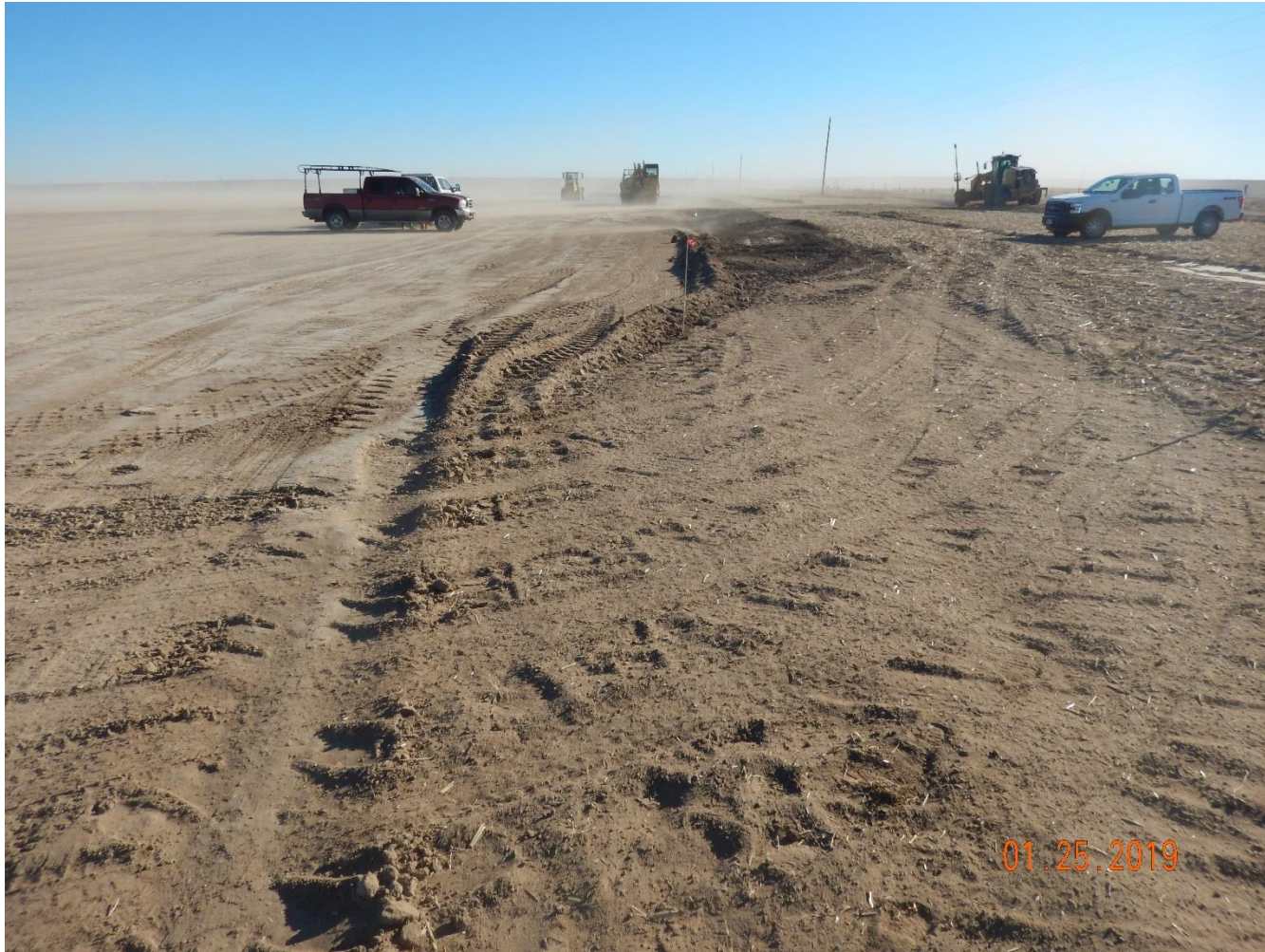
Photo 11: Photo taken from the southwest corner of the pad. Operator appears to have constructed a ditch along the northern end (with exception to the northeast corner), the eastern and southeastern areas of the constructed pad. Photo shows area of the pad on the southwest where the ditch ends. Required stormwater and erosion control BMPs do not appear to have been installed (or constructed in accordance with good engineering practices) along the western, northwest and northeastern areas of the constructed pad. See photos 12
