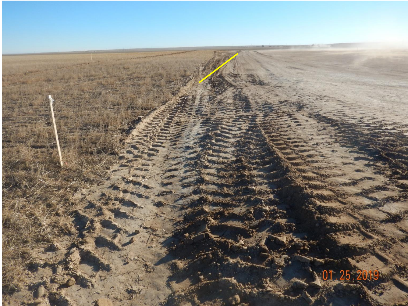
Photo 18: Photo taken from the northwest corner of the pad, facing east. Sufficient stormwater and erosion control BMPs do not appear to have been installed on the northwest corner of the pad. See comments under photo 11. Photo also shows areas where a ditch appears to have been constructed on the north end of the pad.
