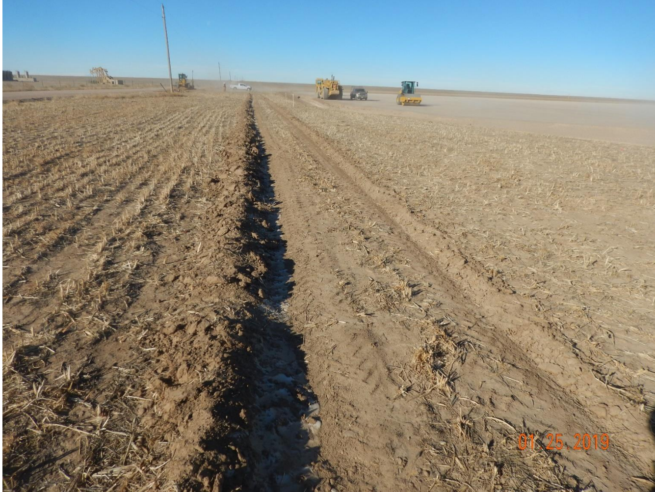
Photo 9: Photo taken from the southeast corner of the location, facing west. Photo shows ditch/berm BMP along perimeter of the location. See comments under photo 2.
