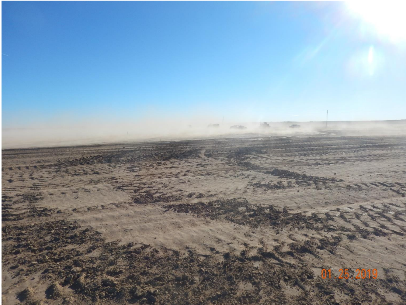
Photo 37: Photo taken from the west end of the location, facing southeast. Photo shows wind erosion transporting sediment offsite. This does not comport with rule 1002.e and 1002.f
