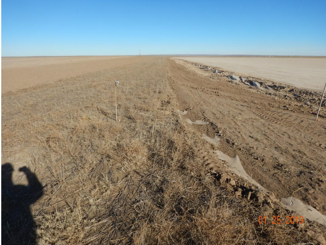
Photo 19: Photo taken from the southwest end of the pad, facing north. Photo shows stormwater and erosion control BMPs do not appear to have been installed in accordance with good engineering practices, and is insufficient. See comments under photo 11.
