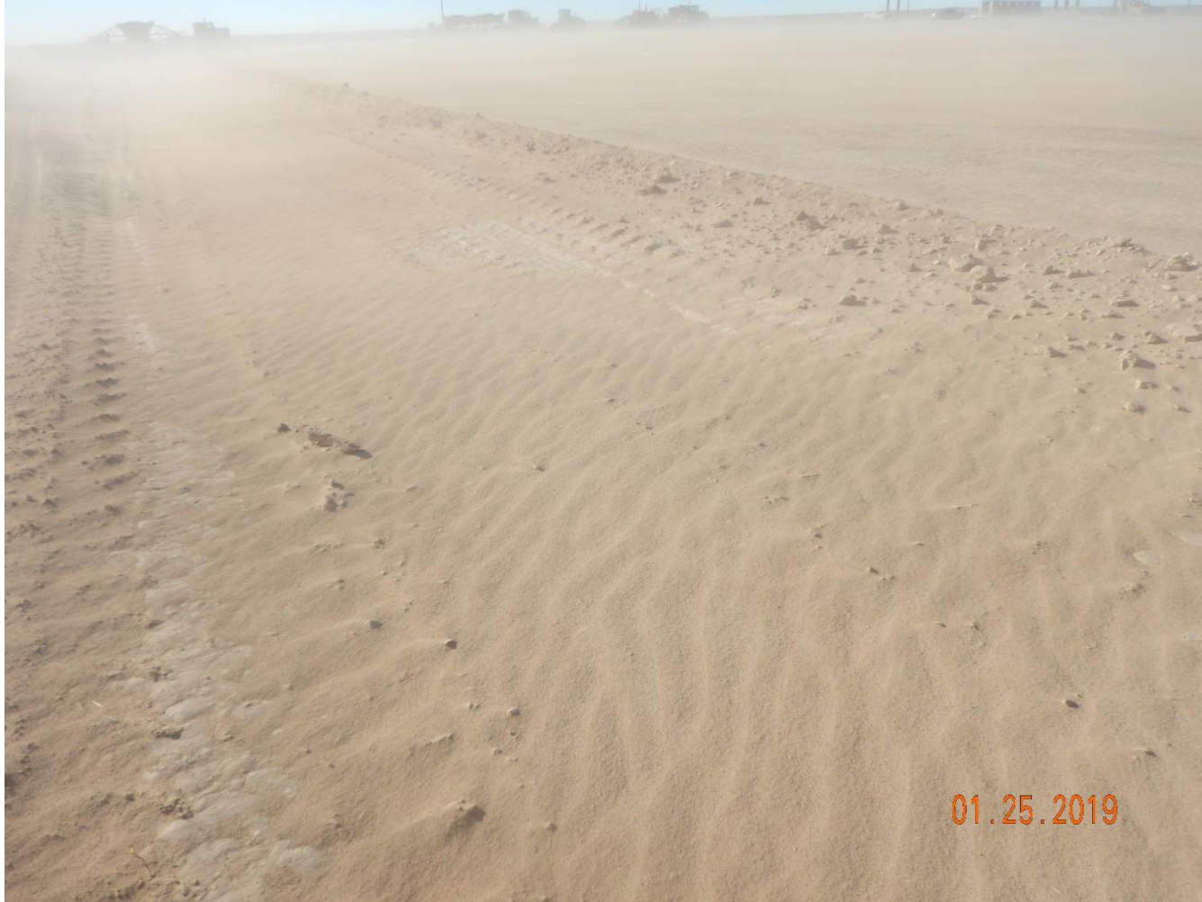
Photo 38: Photo taken from the stormwater ditch on the east end of the location. Photo shows sediment deposition due to wind erosion within the ditch.
