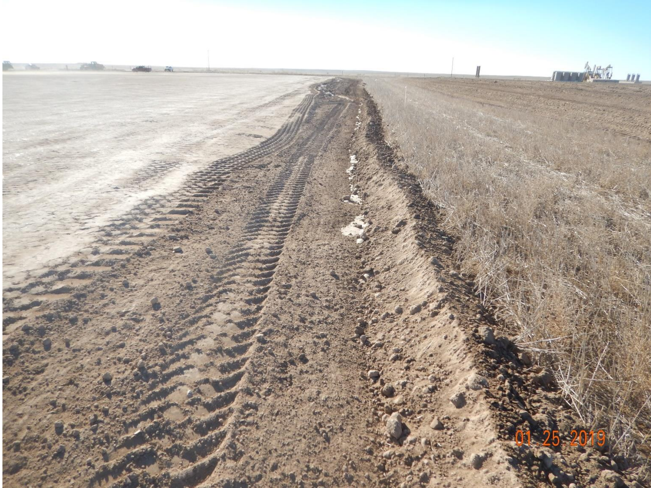
Photo 15: Photo taken from the west end of the pad, facing south. Photo shows stormwater and erosion control BMPs do not appear to have been installed in accordance with good engineering practices, and is insufficient. See comments under photo 11.
