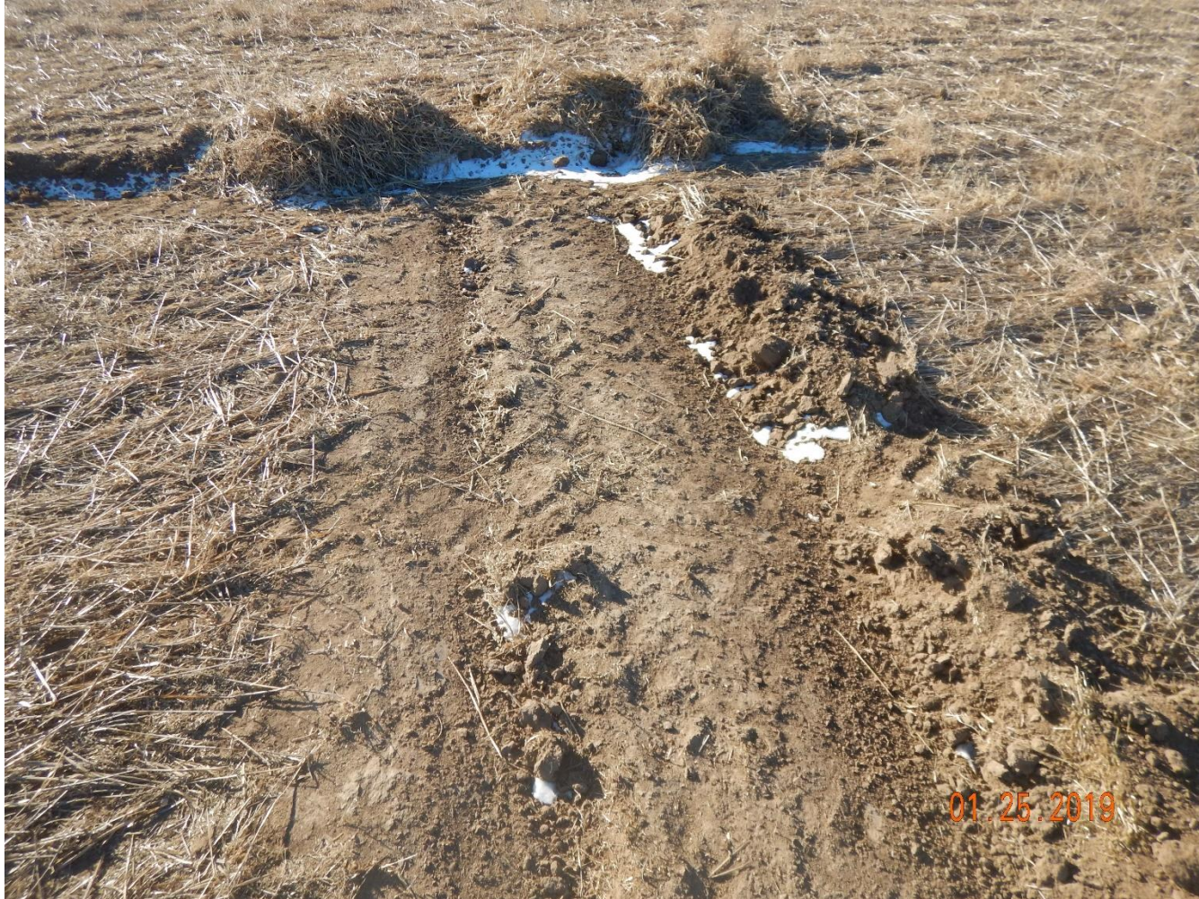
Photo 4: Photo taken from the southwest corner of the location. Photo shows ditch/berm BMP along perimeter of the location. See comments under photo 2.
