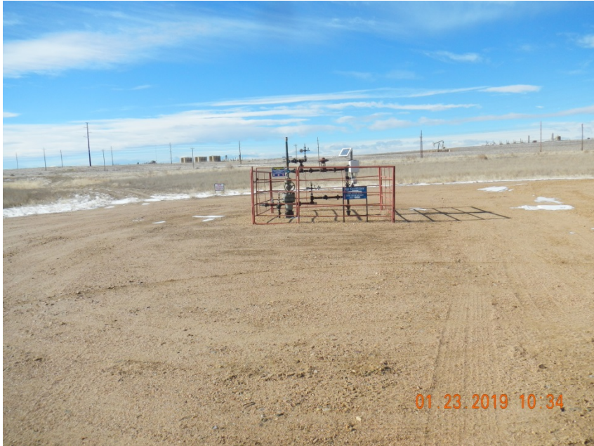
Photo 1. Photo taken from the location, facing Southwest. Appears the Operator has removed all well equipment from the P&A well on the Active Location.
