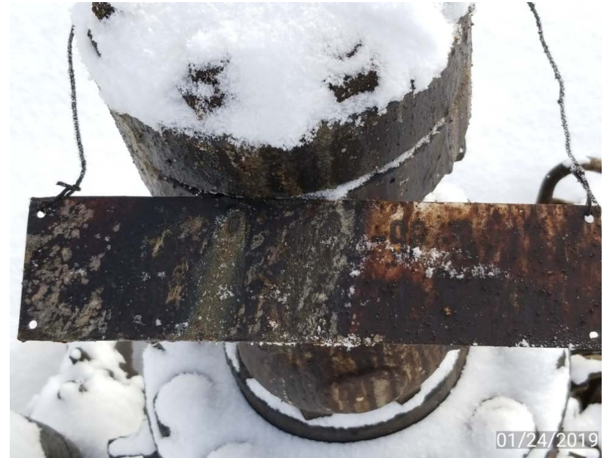
Photo 2. Well head sign not legible.
