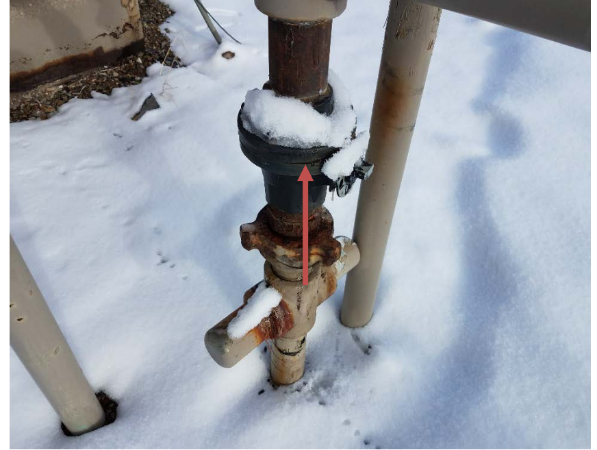
Location Photo #2, small leak noted on this valve.
