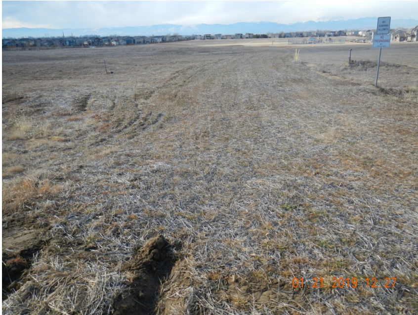
Photo 1. Photo taken from the access road of CR 7, facing West. Appears the Operator has performed final reclamation activities with the evidence of drilling rows and straw crimped mulch.
