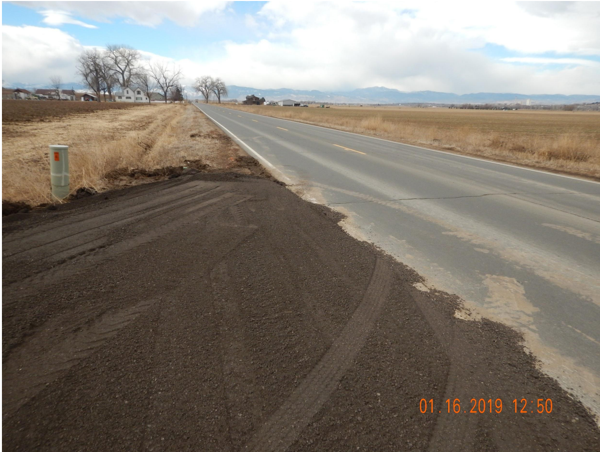
Photo 4. Photo taken from the entrance of location, facing West. Photo illustrates there is no vehicle track out issues. Operator is still constructing the access road and has additional vehicle tracking device BMPs planned.
