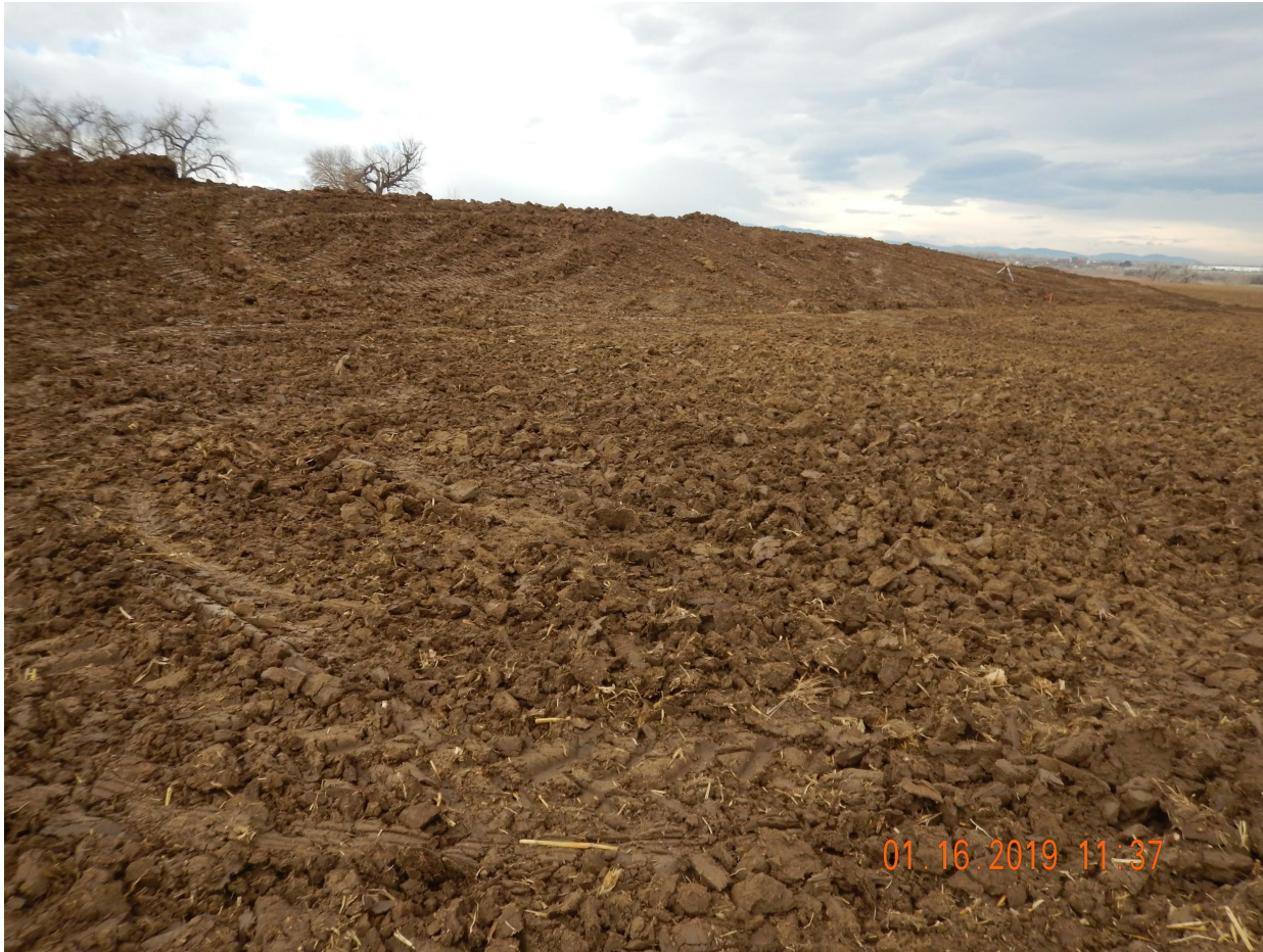
Photo 1. Photo taken from the western location, facing Northwest. Photo illustrates the western topsoil stockpile. Operator was still salvaging topsoil from the northern location. Based on field observations, it appears the Operator is salvaging all topsoil from disturbance areas.
