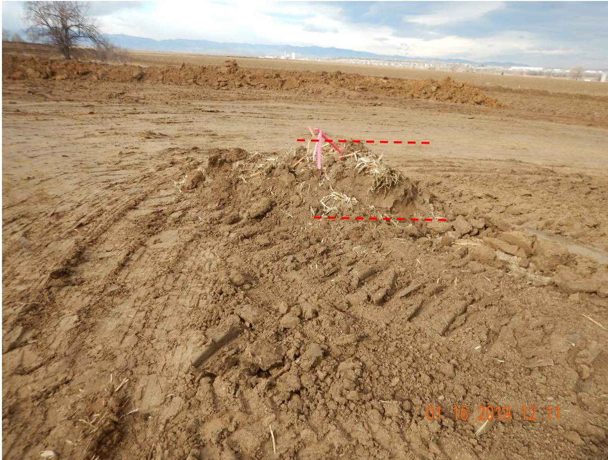
Photo 3. Photo taken from the central location, facing Northwest. Photo illustrates the original surface height compared to how much topsoil is being salvaged. Appears about 15" of topsoil has been salvaged from the location.
