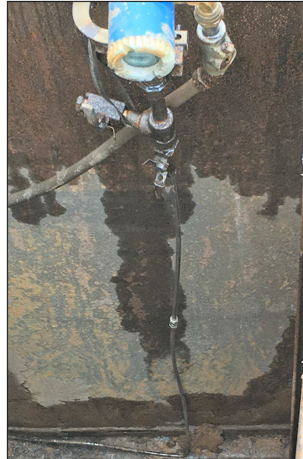
3/8" Stainless steel process piping that separated and was point of release. Line repaired in picture with coupler
