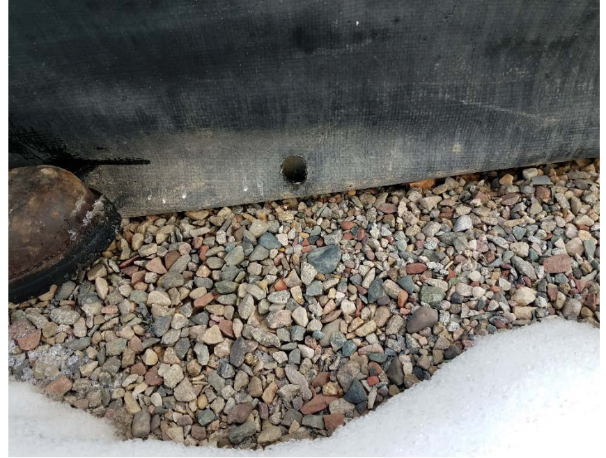
Location Photo #4, Hole in secondary containment liner.
