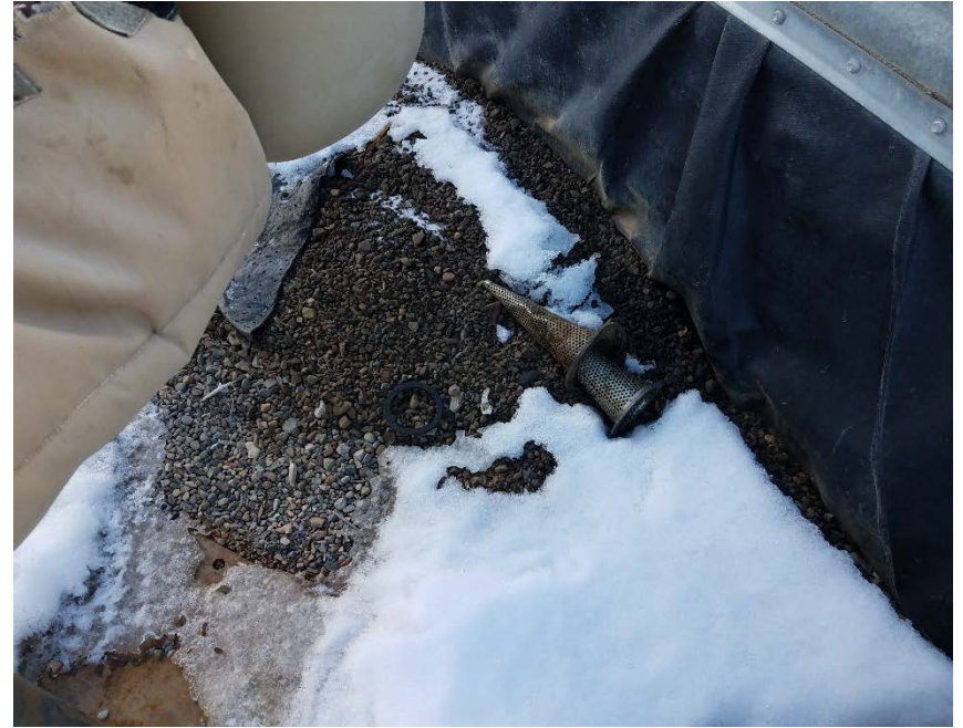
Location Photo #4, , Stained ground in battery containment near load out point.
