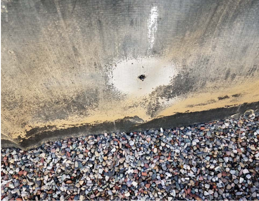
Location Photo #9, Holes in containment secondary liner.
