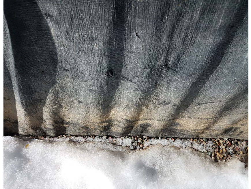
Location Photo #10, Holes in containment secondary liner.
