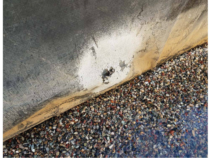
Location Photo #4, Holes in secondary containment liner.
