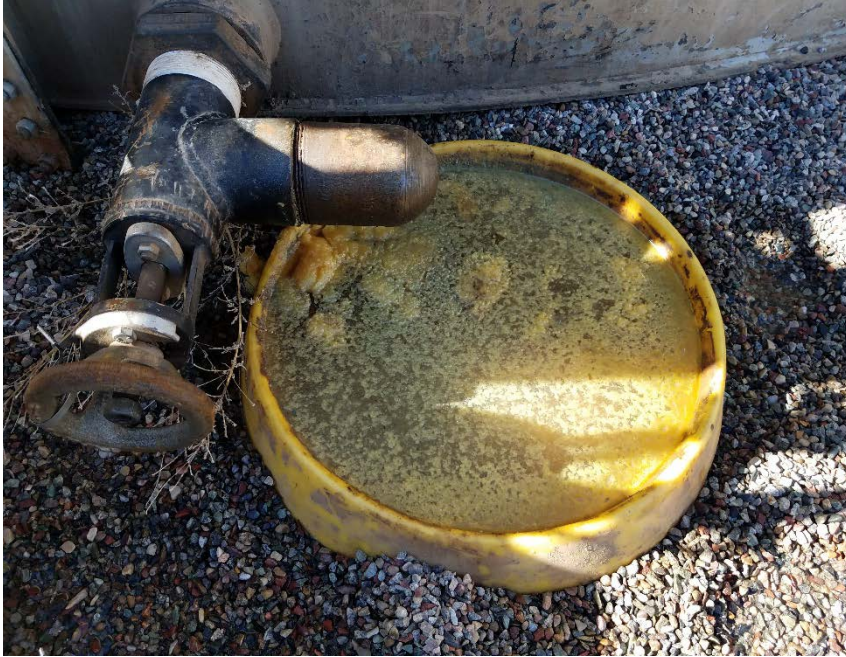
Location Photo #3, Condensate in drip pan.
