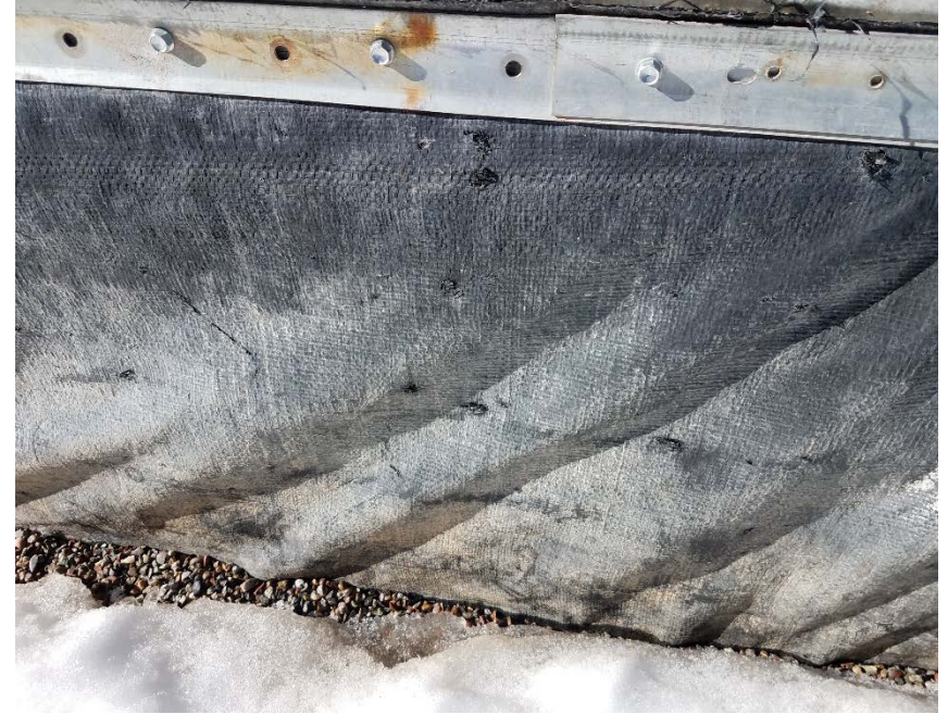
Location Photo #6, Holes in secondary containment liner.
