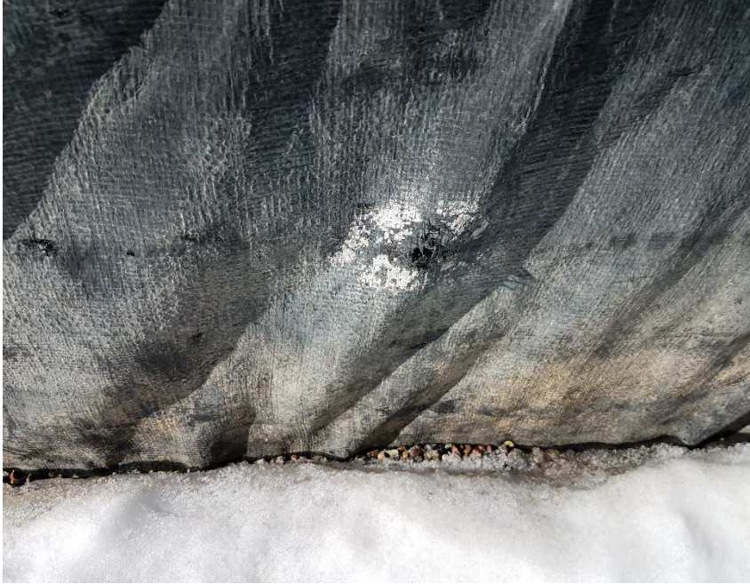
Location Photo #5, Holes in secondary containment liner.
