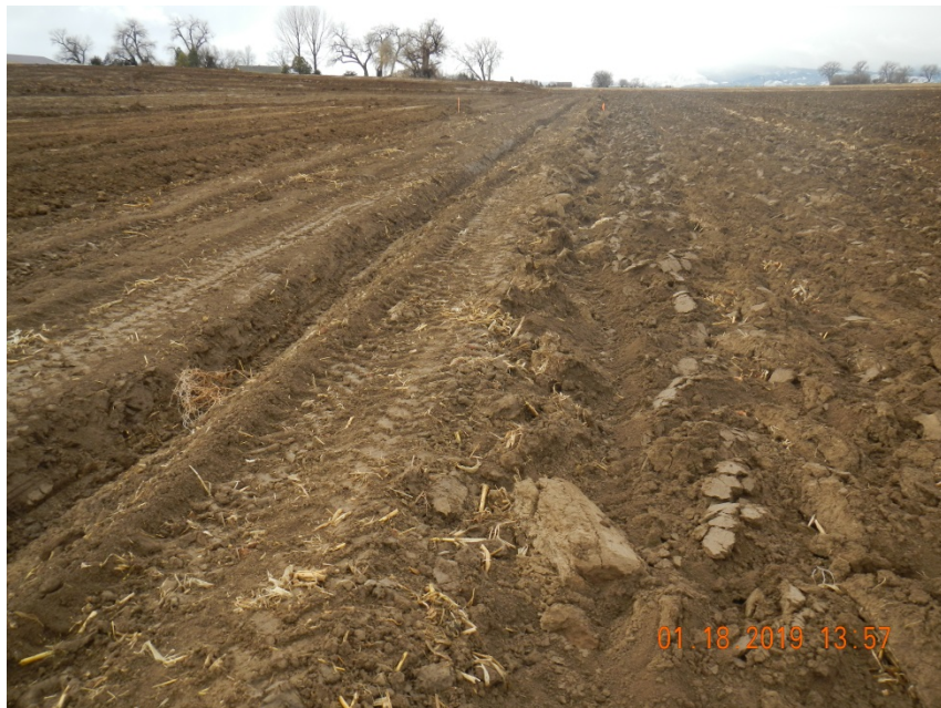
Photo 5. Photo taken from the northern perimeter of the location, facing West. Photo illustrates the ditch and berm BMP that has been installed around the perimeter of the location.
