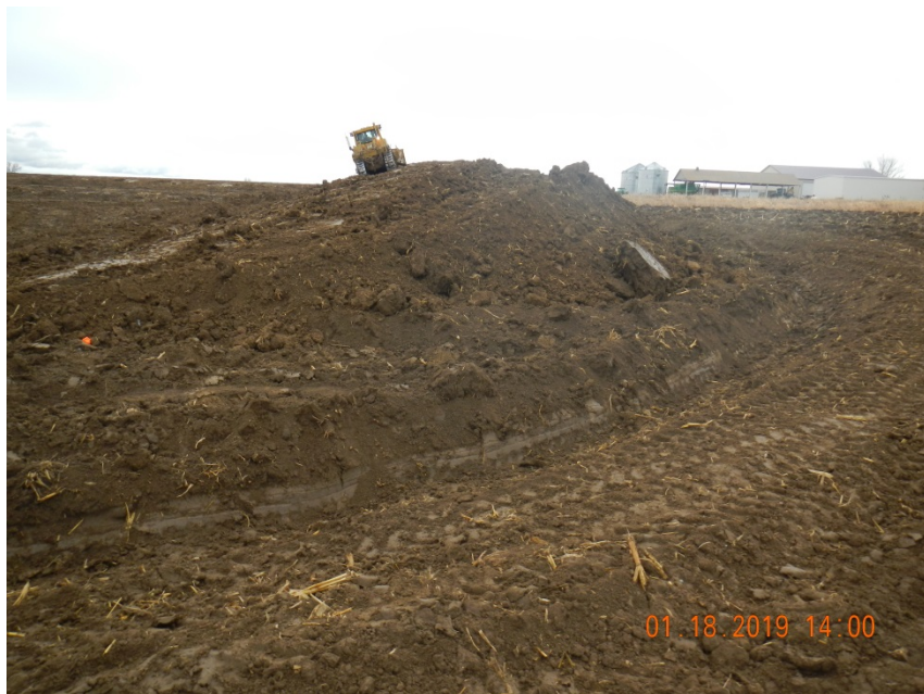
Photo 7. Photo taken from the northwestern perimeter of the location, facing South. The topsoil stockpile being stored along the eastern area has been temporarily stabilized with equipment tracking.
