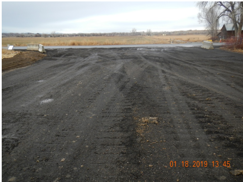
Photo 1. Photo taken from the entrance of the location off CR 205, facing North. Operator has installed gravel potentially to limit tracking onto the county road. BMPs in proper functioning condition at the time of this inspection.
