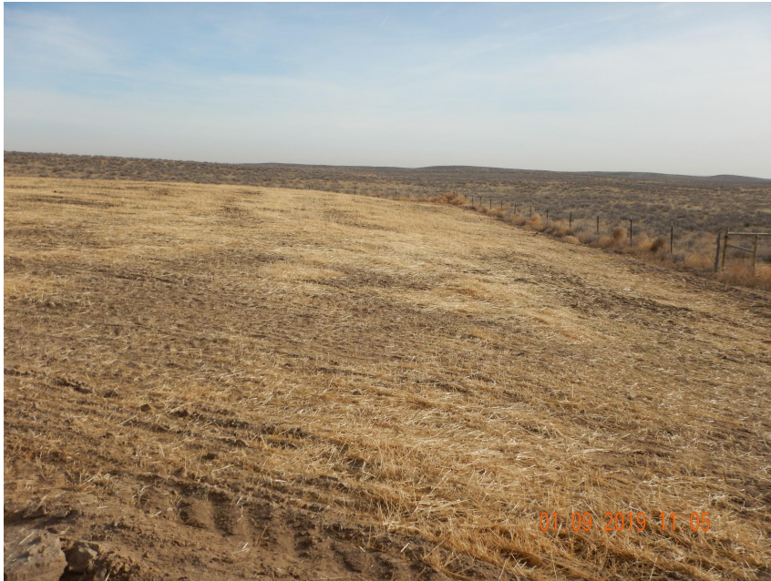
Photo 3. Photo taken from the southeast location, facing East. Operator has performed interim reclamation activities with the evidence of drilling rows and straw crimped mulch. However, interim areas do not appear to be properly contoured to the surrounding landscape- see Photos 5 & 6.
