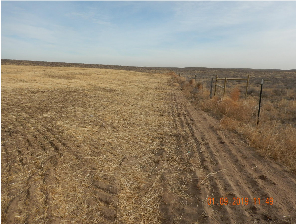
Photo 5. Photo taken from the southern perimeter of the location, facing East. Photo illustrates interim areas do not appear to be properly contoured to the surrounding landscape. Further review is required but Operator may need to perform additional contouring to comply with Rule 1003 standards.
