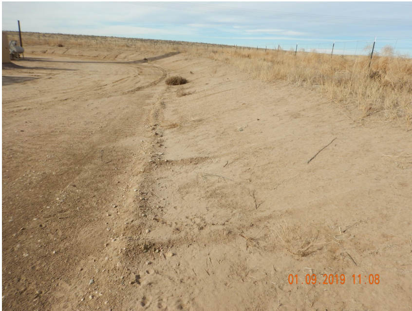
Photo 9. Photo taken from the northern location, facing West. Tackifier was observed on the cut slope but appears to be in need of maintenance.
