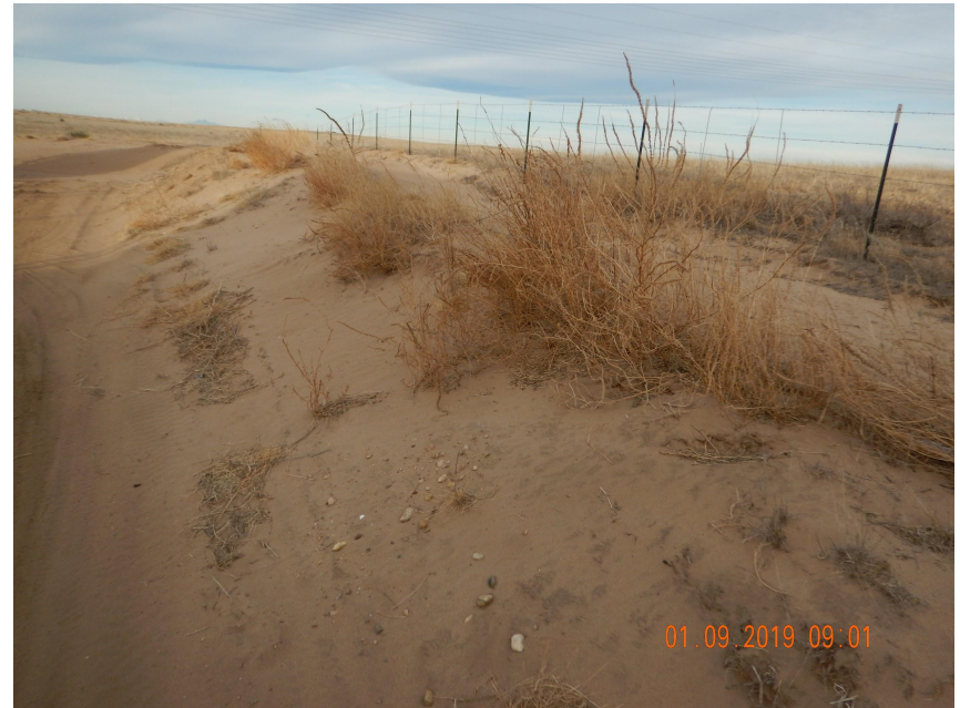
Photo 6. Photo taken from the northern location, facing West. Cut slope is not stabilized.
