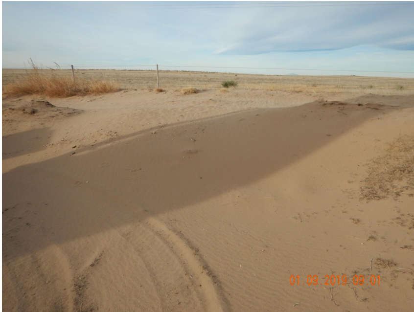
Photo 7. Photo taken from the northwestern location, facing West. Site degradation is occurring due to the lack of stabilization along the cut slope.
