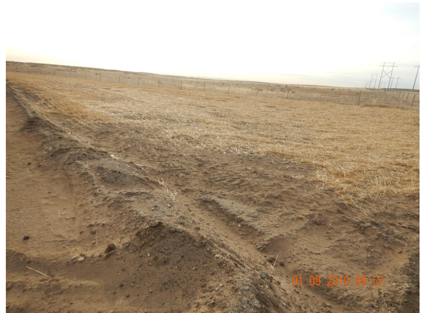
Photo 2. Photo taken from the southwest location, facing Southeast. Operator has performed interim reclamation activities with the evidence of drilling rows and straw crimped mulch. Interim areas appear to be properly contoured to the surrounding landscape.
