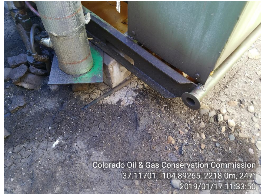
PHOTO 4: STAINED SOIL NEAR ENGINE SKID
