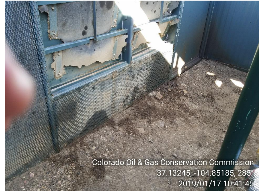
PHOTO 4: STAINED SOIL INSIDE SOUND WALL AROUND COMPRESSOR
