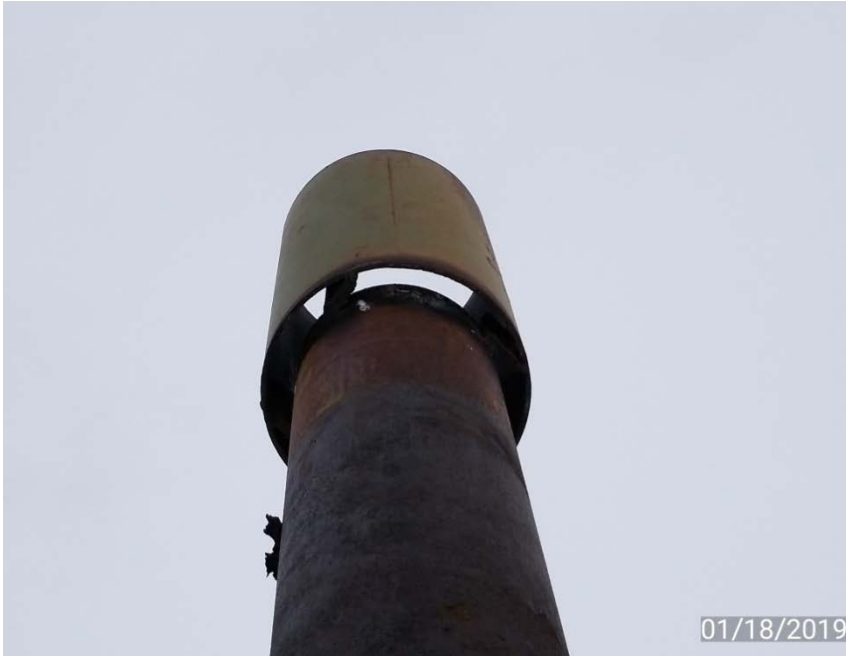
Photo 3. Separator vent stack without bird protection.
