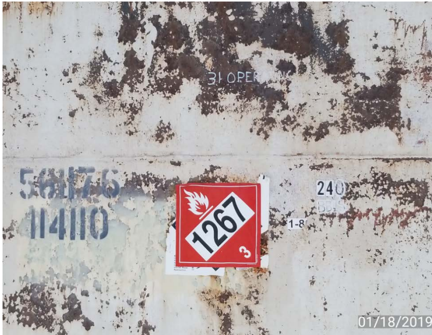
Photo 3. Tank missing NFPA label. Operator displayed as "31 Operating".
