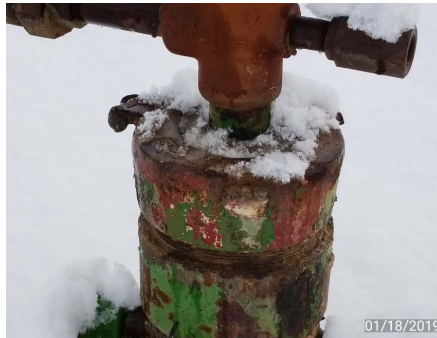
Photo 2. Well head leaking gas.
