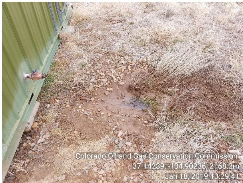
Photo 3 stained soil under 1" drain line for separator
