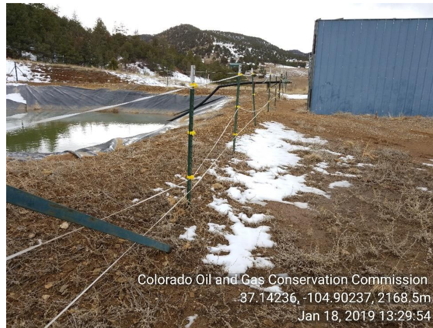
Photo 4 Electric fence around lined pit in disrepair
