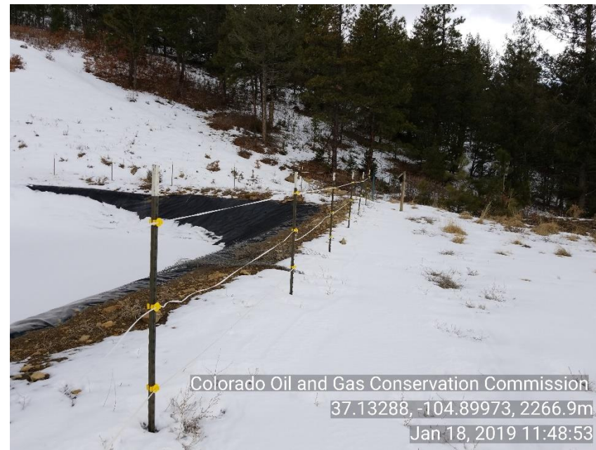
Photo 6 electric fence around lined pit in disrepair
