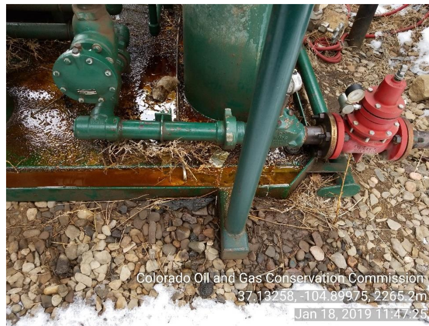
Photo 4 Stained soil and fluid dripping out of liquid ring skid
