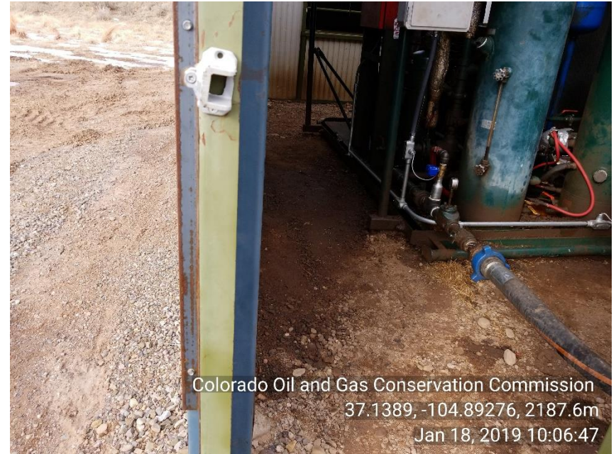
Photo 6 Stained soil around liquid ring skid
