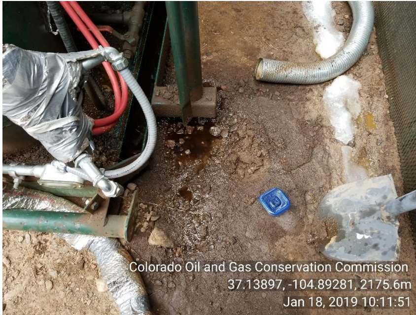
Photo 9 stained soil around liquid ring skid took soil sample
