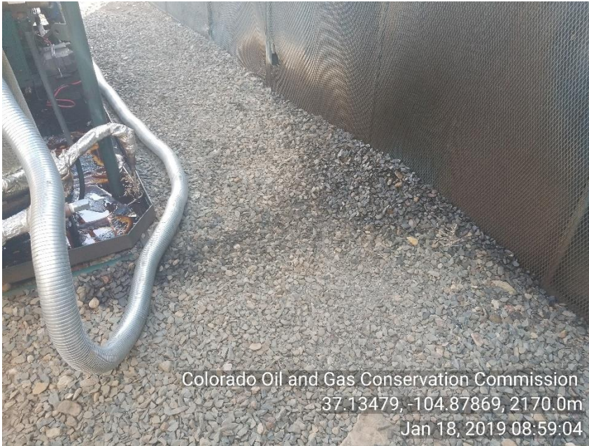
Photo 5 Stained soil around base of liquid ring skid
