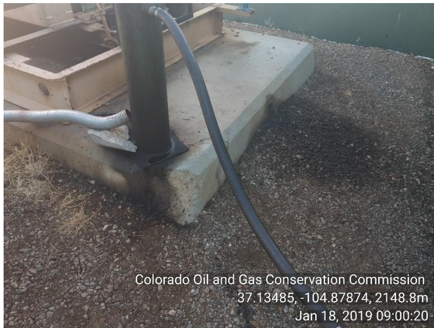
Photo 3 Stained soil around cement base of PU
