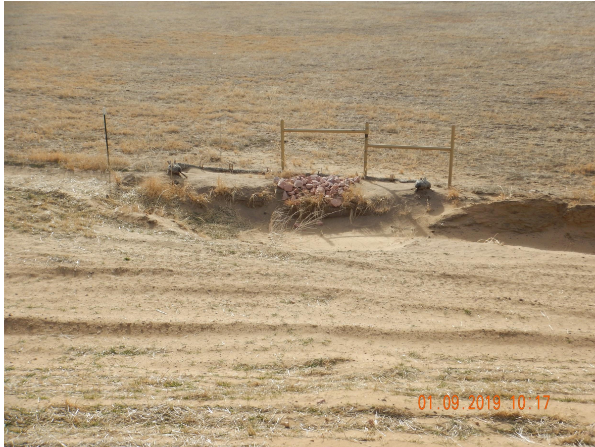
Photo 10. Photo taken from the southern well pad, facing South. Photo illustrates a sediment trap that has not been implemented in accordance with good engineering practices, has not been maintained to properly function, and does not appear to be adequately sized.
