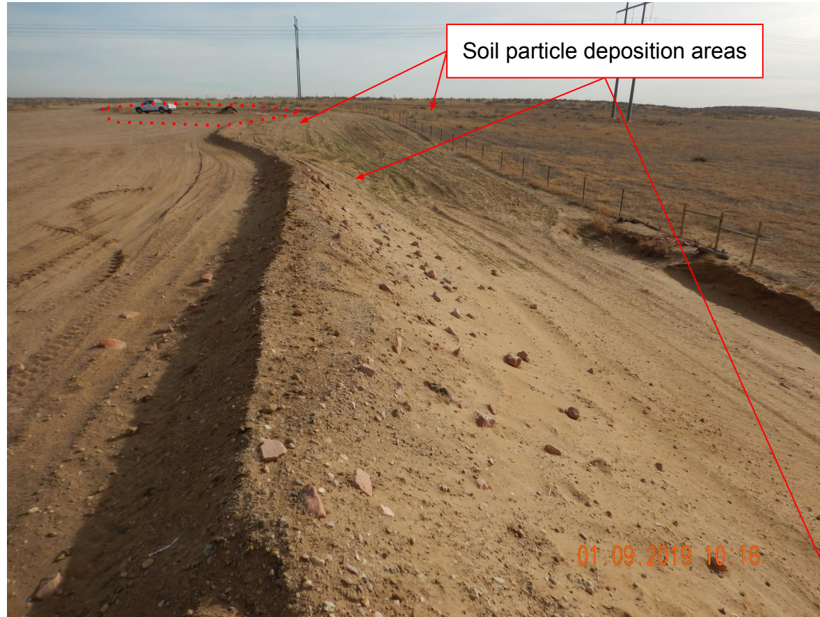
Photo 9. Photo taken from the southwestern well pad, facing East. The red-dotted circle indicates the area that does not appear to be needed for production operations and shall be reclaimed per Rule 1003. Also, appears this portion of the well pad and perimeter are not adequately stabilized, further support for reclaiming the area and implement long-term stabilization through revegetation. See Photos 11-13.
