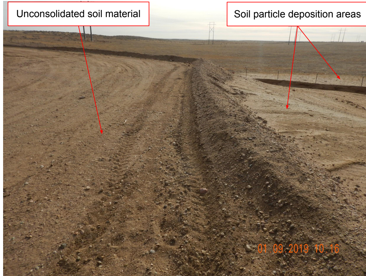
Photo 4. Photo taken from the southwestern well pad, facing South. It appears unconsolidated soil material from the well pad has not been adequately stabilized to control dust and wind erosion. Photo illustrates soil particle deposition as a result of wind erosion onto fill slopes and along the southwestern area off Location.
