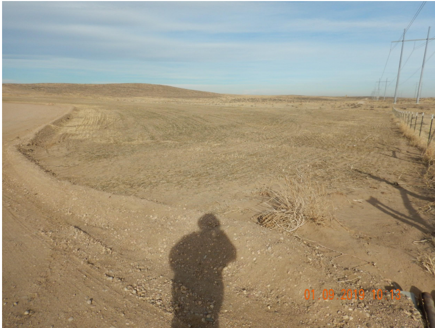
Photo 2. Photo taken from the entrance of the location, facing North. Operator has performed interim reclamation activities with the evidence of drilling rows, straw crimped mulch and germination. Interim areas appear to be properly contoured to the surrounding landscape.
