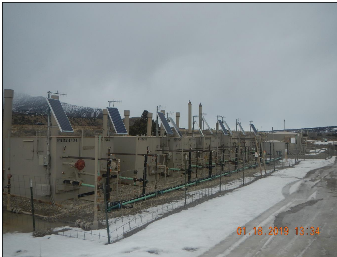
Separators and tank battery.
