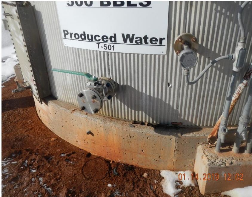
Valve configuration changed to prevent reoccurrence.
