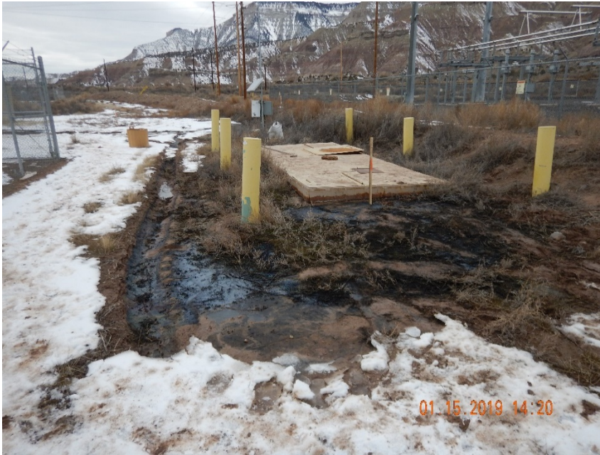
Photo #3 – Stained soil surrounding pipeline vault/POR, looking west.
