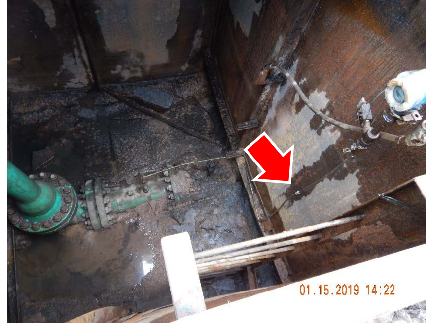
Photo #2 – Looking south into Basin Pipeline WC-4 Vault. Red arrow points to location of 3/8" stainless steel line that was the POR. Stainless steel line had been repaired prior to inspection date.
