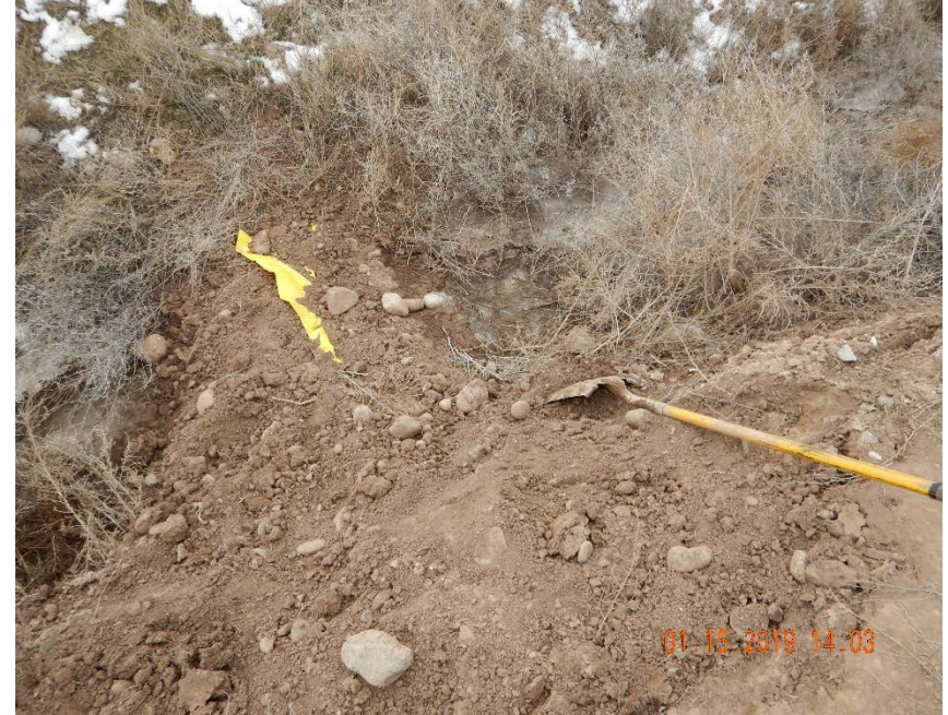
Photo #12 – Earthen dam inside of overflow channel was constructed by operator during initial spill response efforts.
