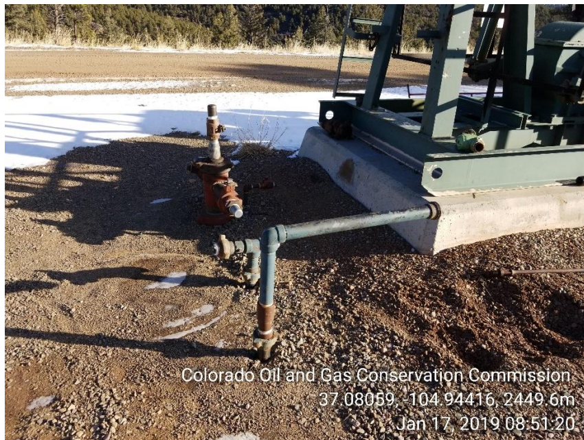
Photo 3 Unmarked, unused and not LOTO risers
