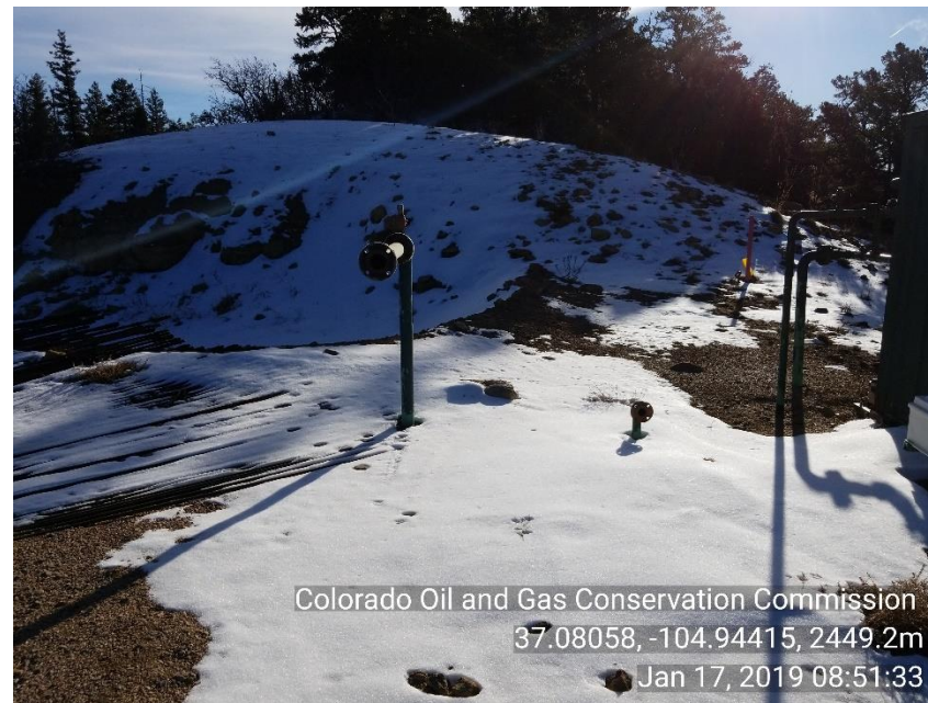
Photo 4 Unmarked, unused and not LOTO risers
