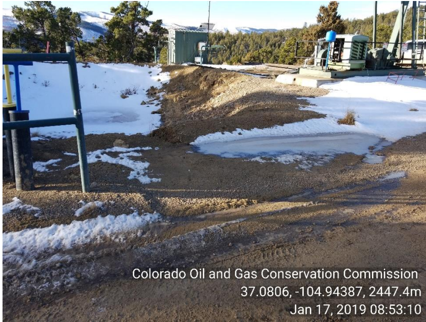
Photo 5 Drainage from road draining into pit
