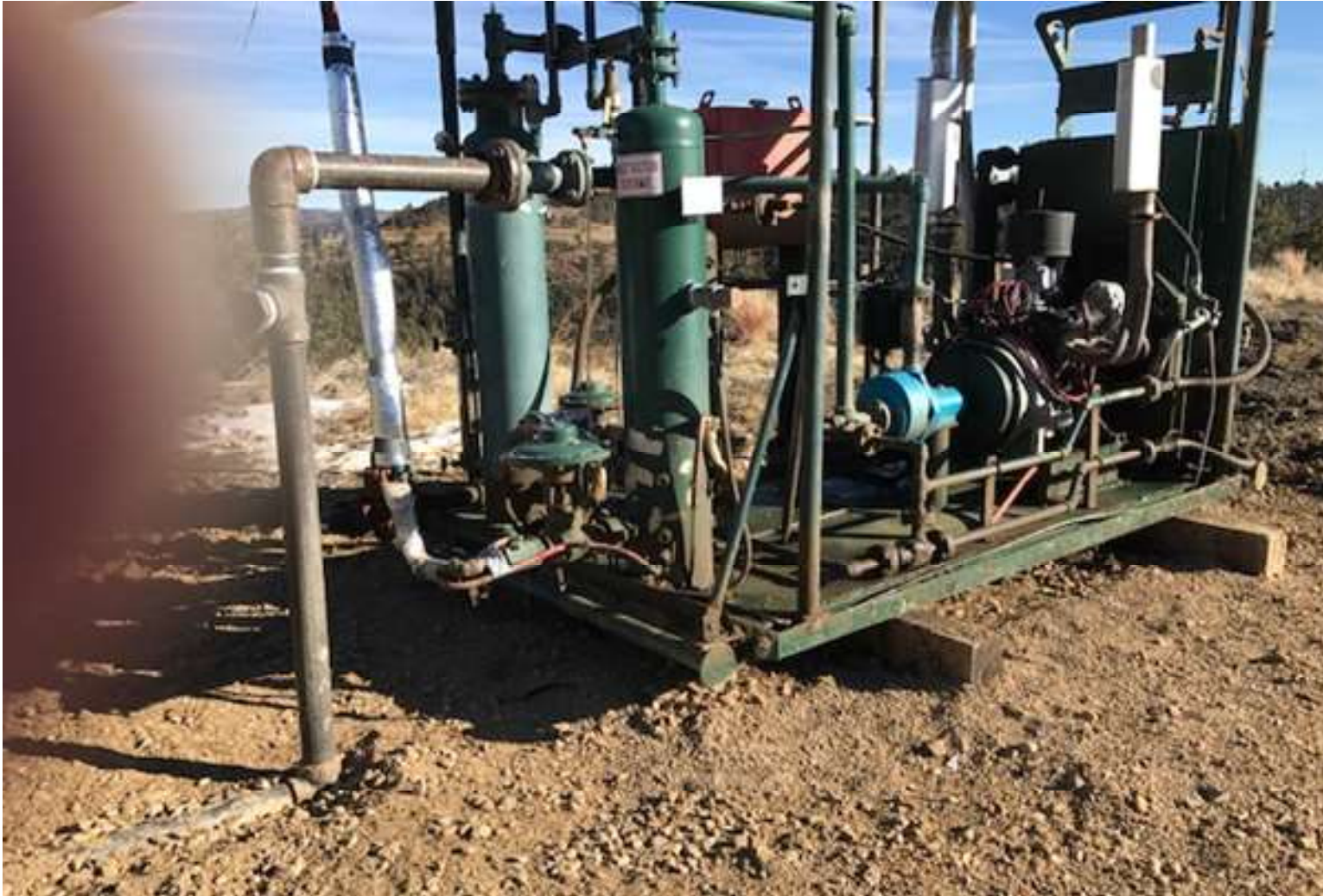
PHOTO 1: THE LIQUID RING COMPRESSOR WAS ELEVATED OFF OF THE GROUND AND THE STAINS WERE REMOVED FROM THE GROUND. ALL VALVES, PIPES AND FITTINGS ARE SECURELY FASTEN TO ENSURE GOOD MECHANICAL CONDITION.
