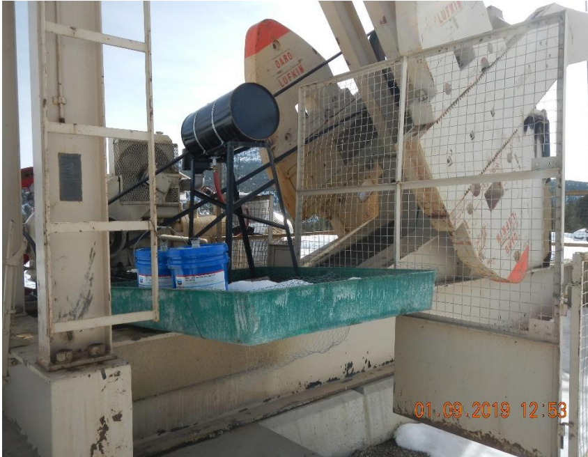
Two five gallon buckets of engine oil stored in secondary containment for lube oil container.
