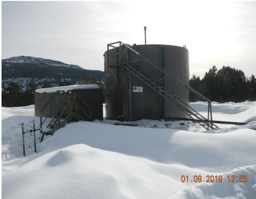
400 bbl. produced water AST installed since last inspection.
