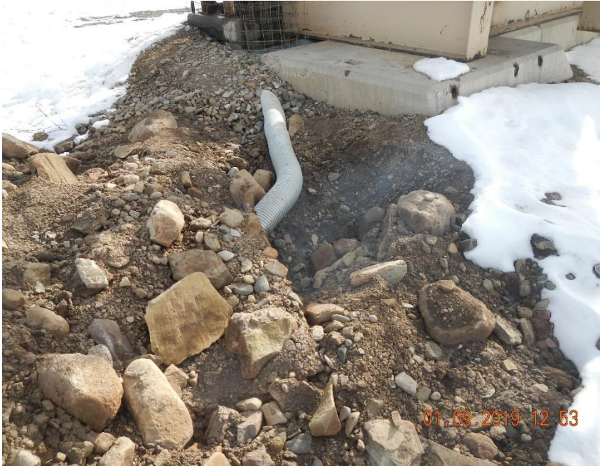
Prime mover exhaust routed underground.
