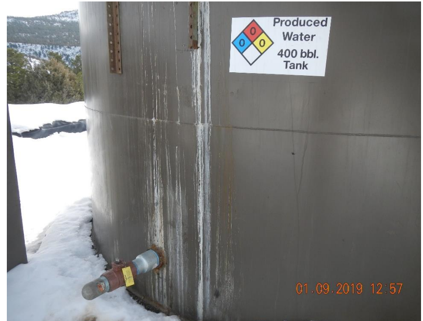
AST is stained and NFPA placard has zeros for all fields.
