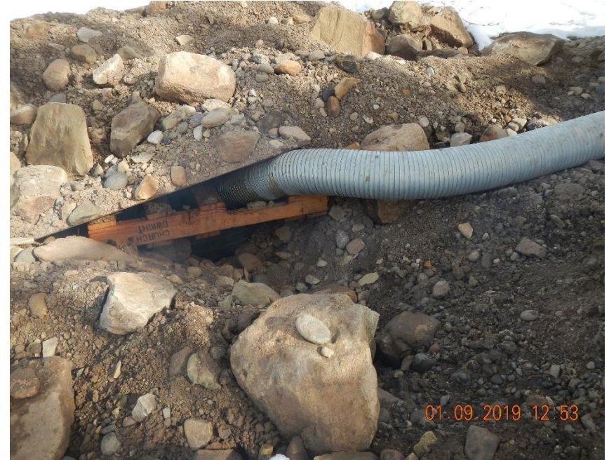
Prime mover exhaust pipe routed underground, reportedly for noise control.
