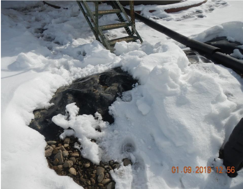
Liner in secondary containment berm for 400 bbl. AST.
