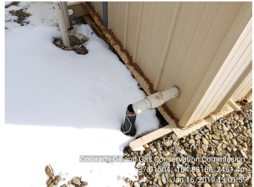
Photo 4 Unmarked and unused riser no LOTO
