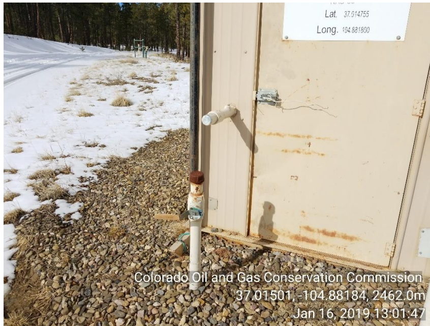
Photo 3 Unmarked and unused riser no LOTO
