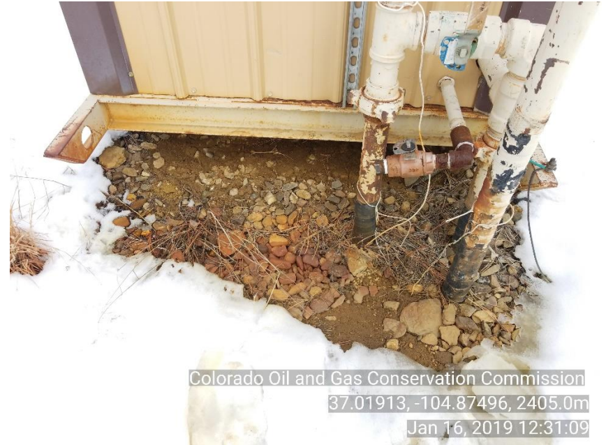
Photo 4 Stained soil by 1" drain line for sep
