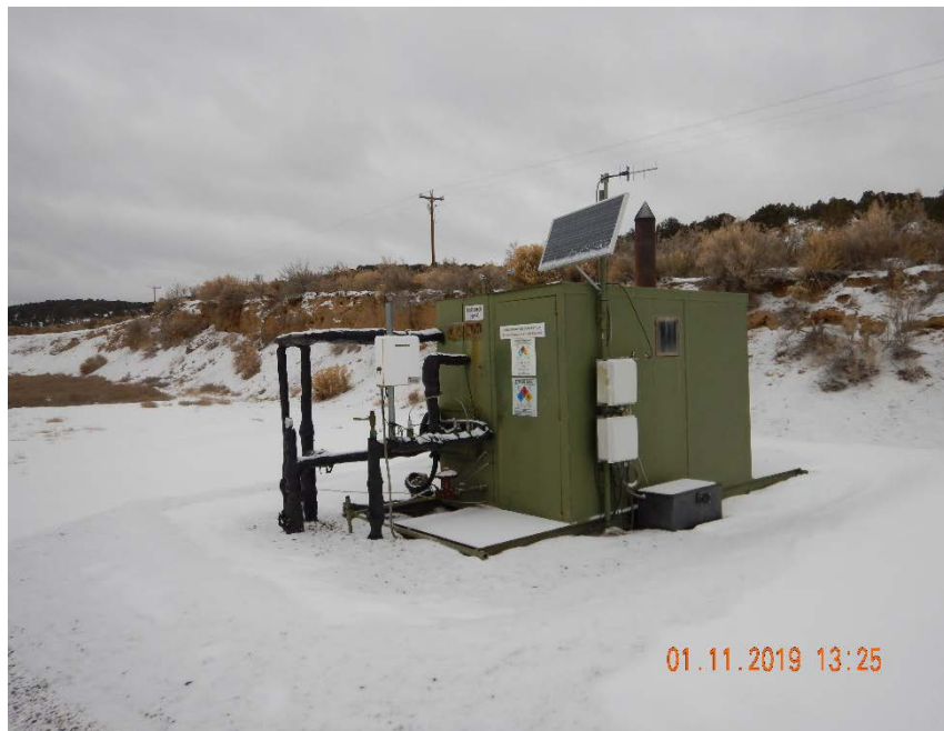
Photo #9 – Horizontal heated separator located on north side of pad.
