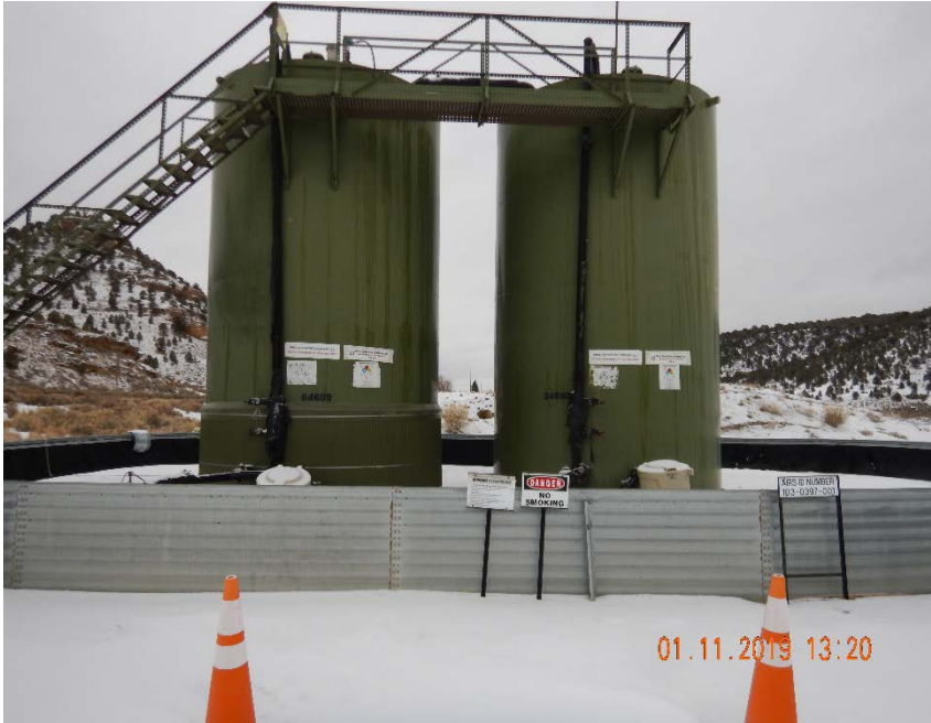
Photo #7 – 400 bbl steel ASTs inside of lined, metal SPCC contain produced water (left tank) and condensate (right tank).
