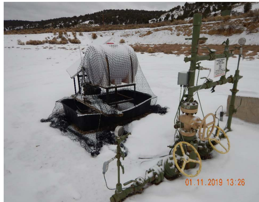
Photo #10 – View of wellhead and day tank with secondary containment device.
