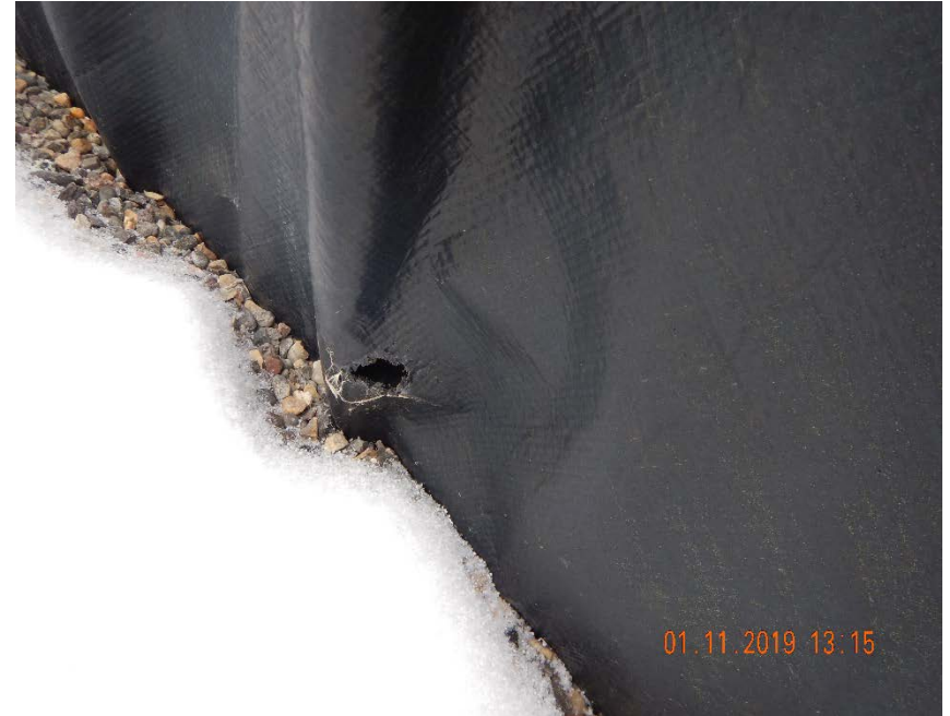
Photo #4 – Small hole in NW corner of metal SPCC liner for 90 bbl produced water AST.
