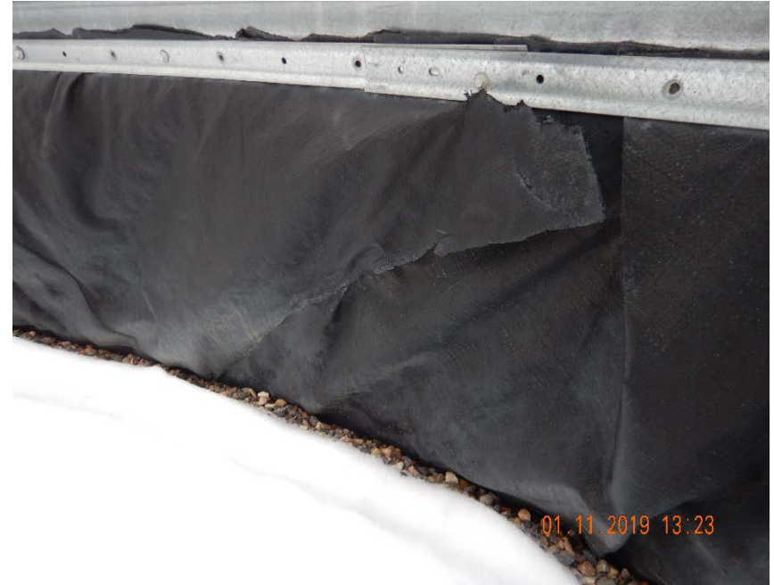
Photo #8 – Tear in liner for 400 bbl ASTs was observed on south end of SPCC.
