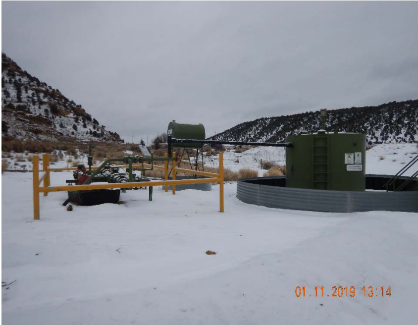
Photo #3 – Pigging station, methanol tank, and 90 bbl produced water AST located at NE corner of pad.
