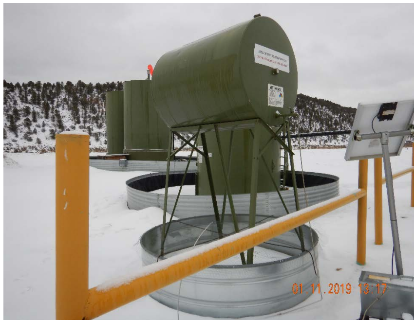
Photo #5 – Methanol tank inside of secondary containment.
