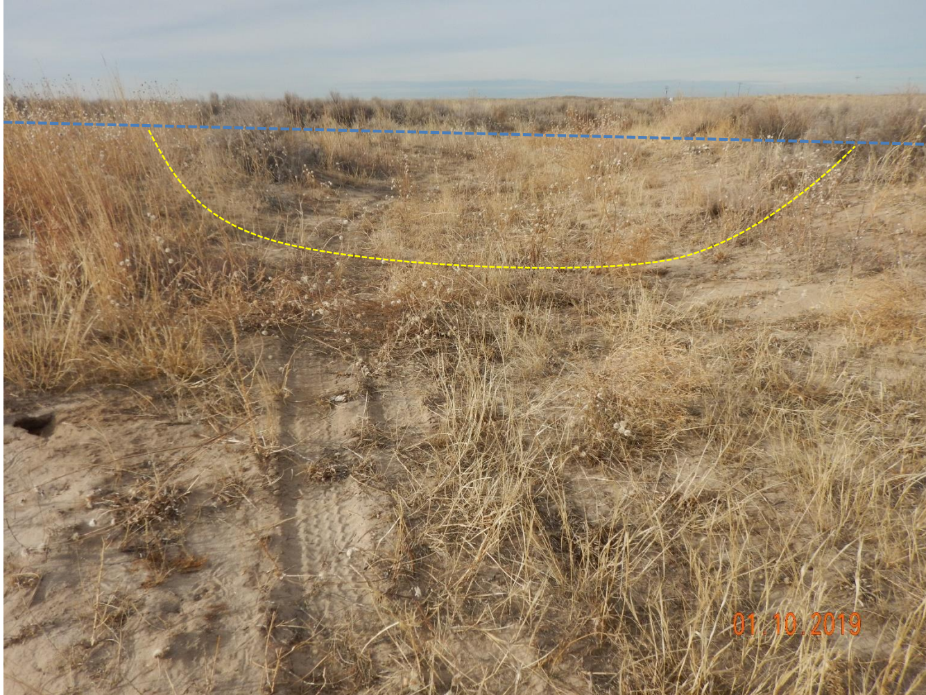
Photo 6: Photo taken from the access road, facing north. Photo shows access road (blue line) has not been recontoured/regraded to that of the adjacent reference area (yellow line)
