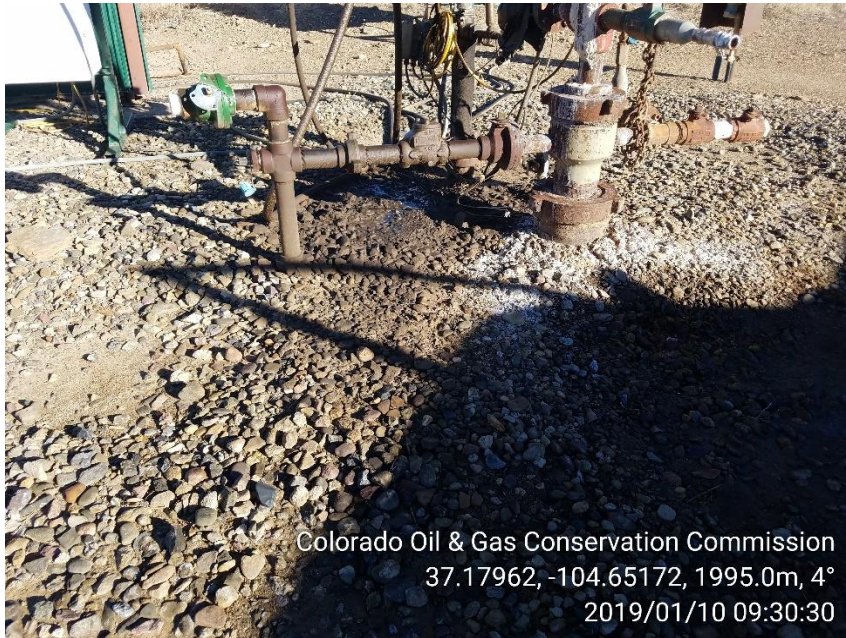
PHOTO 3: STAINED SOIL UNDER DRIVEHEAD MOTOR AROUND WELLHEAD
