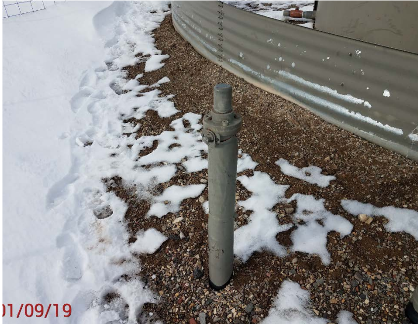
Location Photo #3, unused flow line riser, south end of battery.
