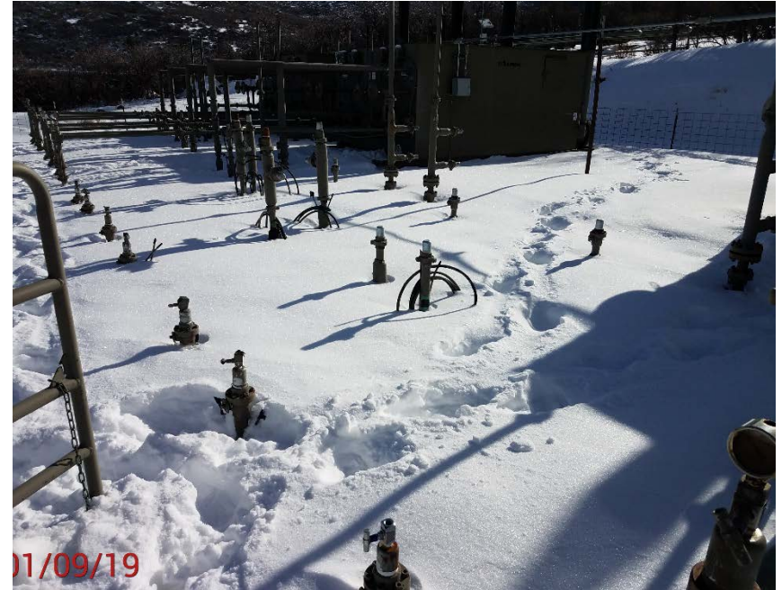
Location Photo #4, Several unmarked flow line risers.
