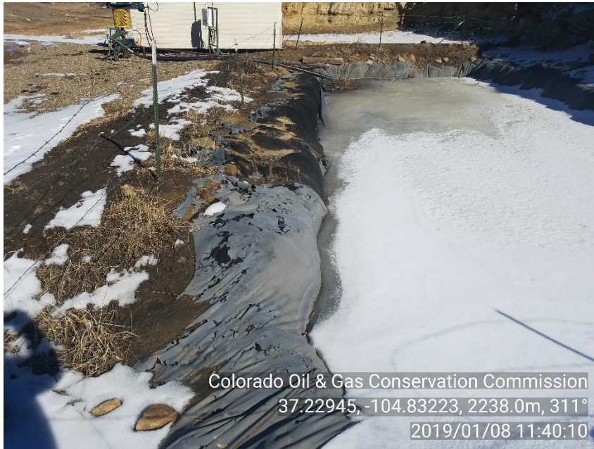
PHOTO 3: LINER TORE AND BREAKING APART
