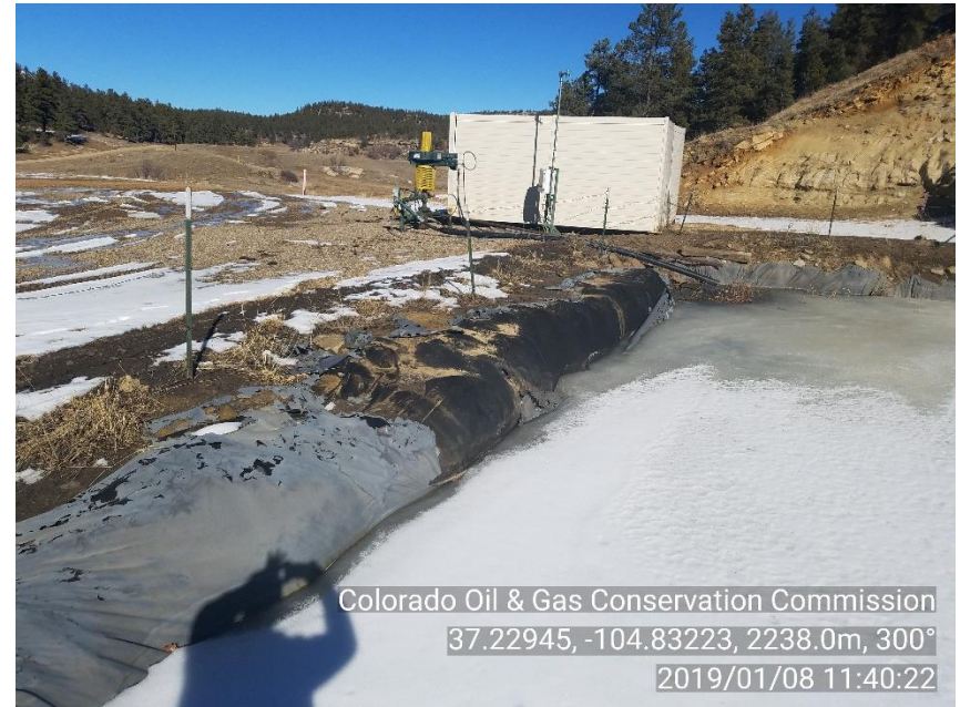
PHOTO 4: LINER TORE AND BREAKING APART
