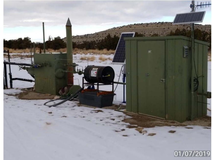
Photo 2. Gas meter building and separator.
